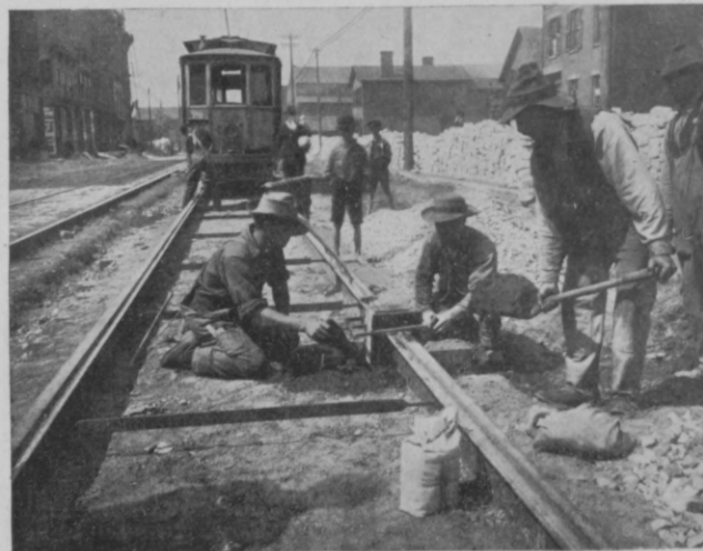
Track Welding in Cleveland.
