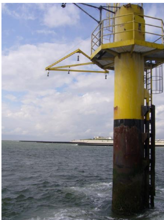
Figure 6: First test assembly at the gauge "Borkum Südstrand". The specially developed triangular extension of the gauge is equipped with four radar liquid-level sensors.
