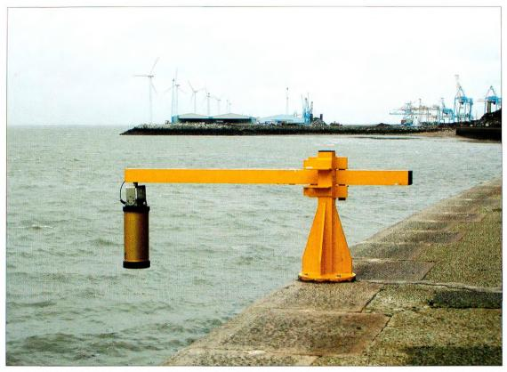
Figure 2: The OTT Kalesto gauge installed at Gladstone Dock, Liverpool
