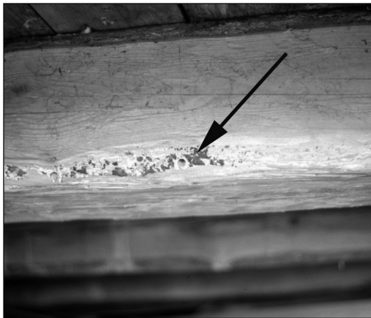
Fig. 4 a boring hole left in a beam illustrated by the arrow. Most boring holes are small (5.1 mm diameter) and so produce no structural issues in the wood.
