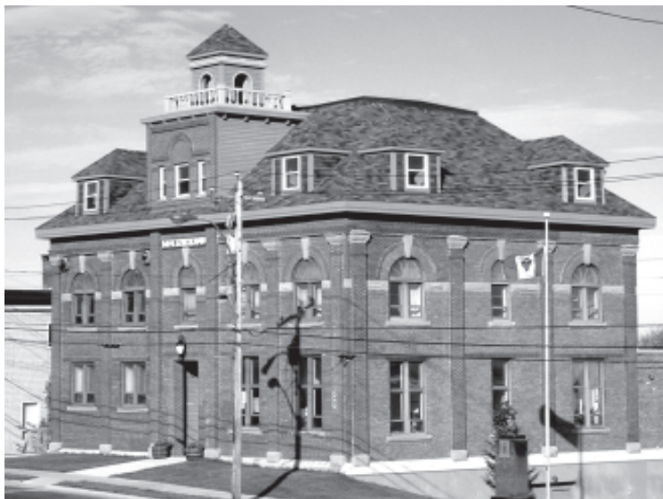
Fig. 2 The elegant, century-old Glace Bay Town Hall, restored recently on the initiative of local volunteers, is now a museum. In 1995, Glace Bay was amalgamated with seven other municipalities to form the Cape Breton Regional Municipality, headquartered in Sydney. Photo: Tom Urbaniak.
