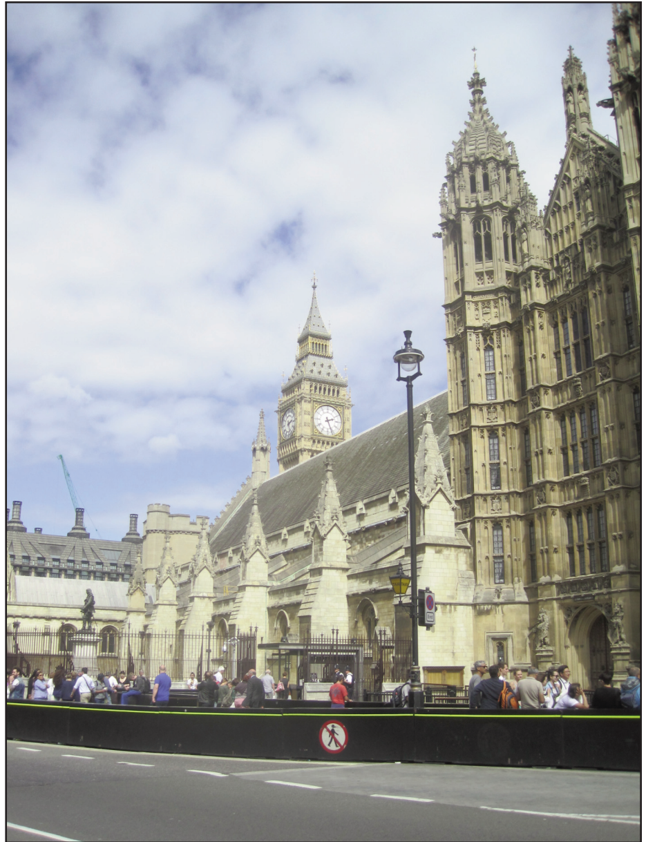
Figure 2. The Palace of Westminster showing pale-coloured Clipsham Stone from recent repairs, contrasting with Clipsham Stone from previous repairs and Anston Stone.
