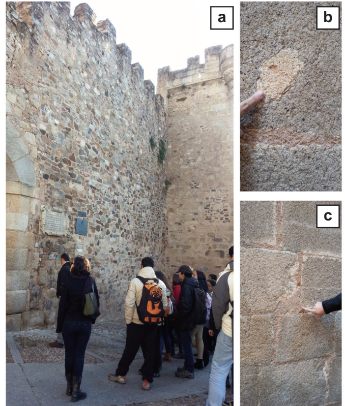
Figure 6. The Roman Wall around the World Heritage City of Cáceres, Spain, and use of mortar that contrasts markedly with the original colour of the granite forming the wall.
