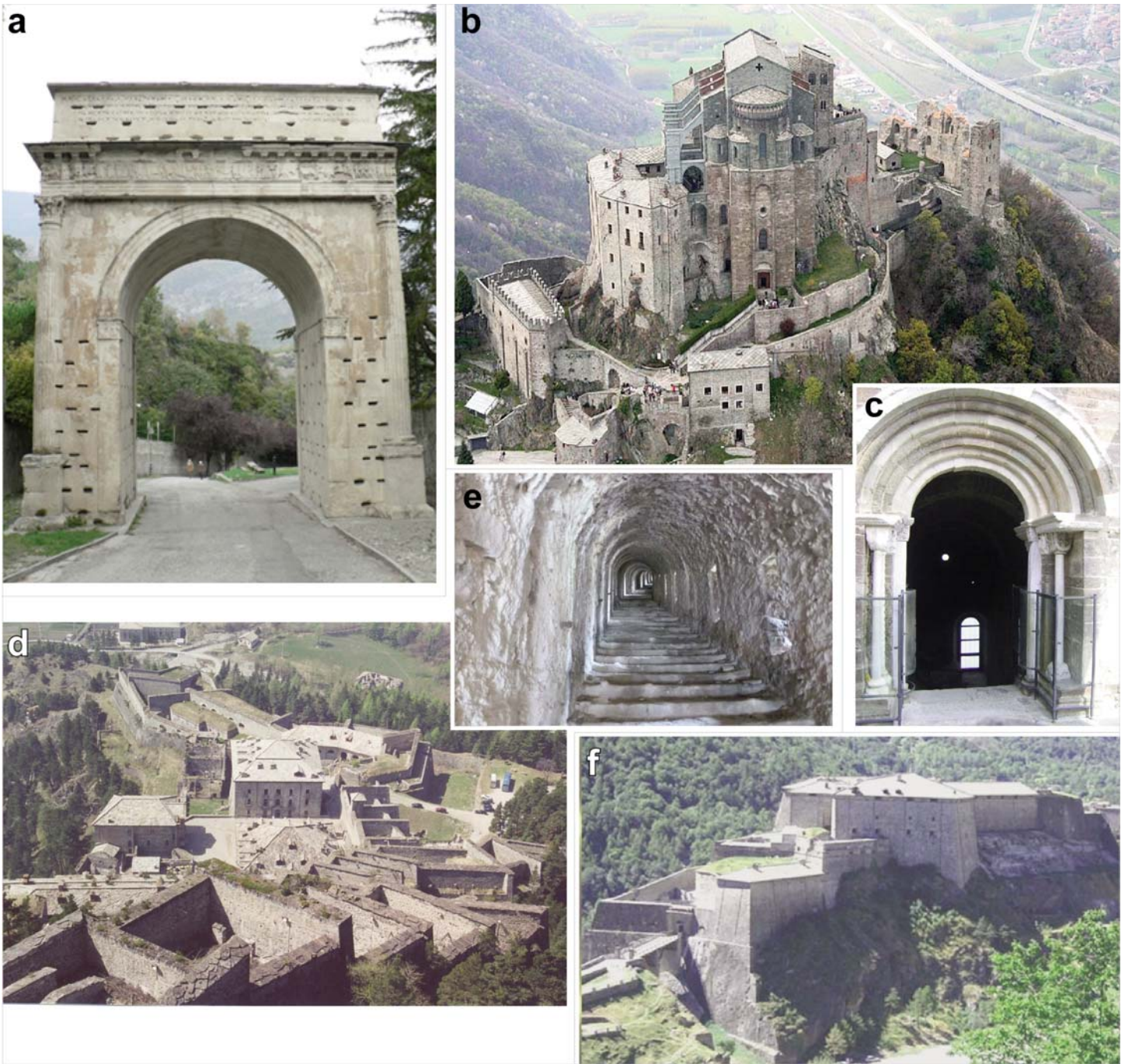
Figure 12. Main examples of employment of Dora-Maira dimension stones in historic buildings: a) Arc of Augustus at Susa (Roman Age, 9 BC); b) Sacra di San Michele Abbey located at the mouth of the Susa Valley; c) ‘Portale dello Zodiaco,’ one of the great expressions of Romanesque art of the 12 th century; d) external features of the Scala Coperta of the Fenestrelle Fortress along the northern slope of the Chisone Valley; e) steps and internal appearance of the Scala Coperta; f) Exilles Fortress located along the Susa Valley.
