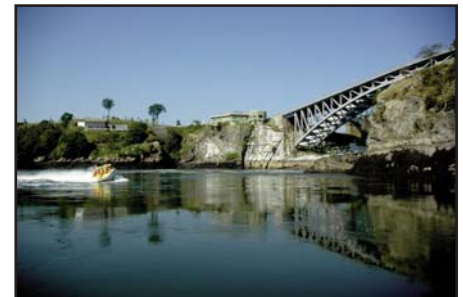
Figure 2. Terrane contact at the Reversing Rapids. Light grey marble of the Neoproterozoic Green Head Group (Brookville Terrane) below the bridge and dark grey shales of the Cambrian-Ordovician Saint John Group (Caledonia Terrane) downriver.
