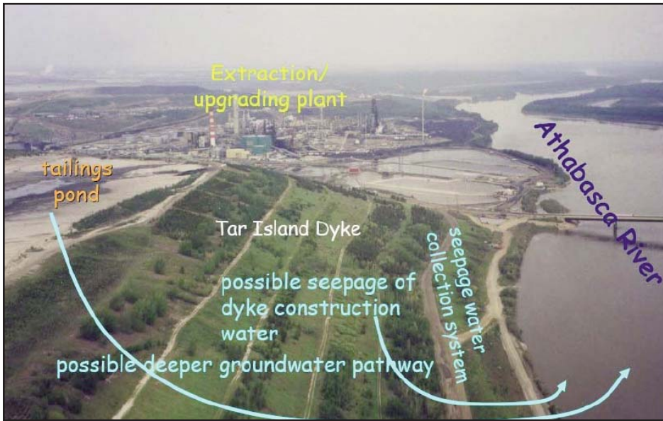
Figure 13. The Tar Island Dyke, looking northward, indicating possible pollution pathways (J.F. Barker, in Royal Society of Canada Expert Panel 2010).
