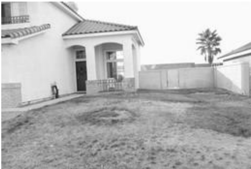
Figure 3: Conversion of a Typical Residential Property From Traditional Lawn to Xeriscape (Before) Southern Nevada Water Authority (2)
