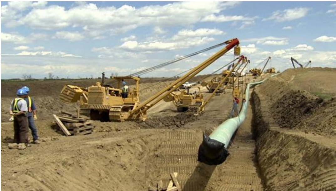
Picture 4: Burying The Keystone XL Pipeline
