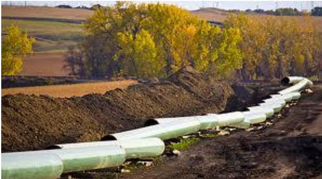
Picture 3: Keystone XL Pipeline Construction – Texas
