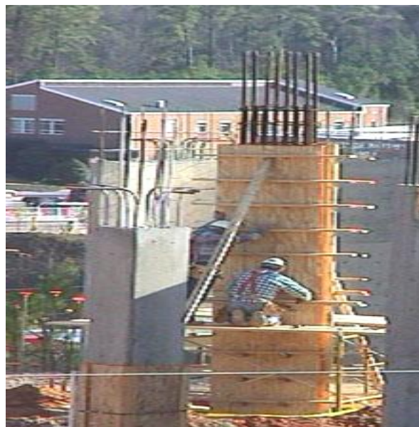
Figure 4: Digital Photograph of Formwork.
