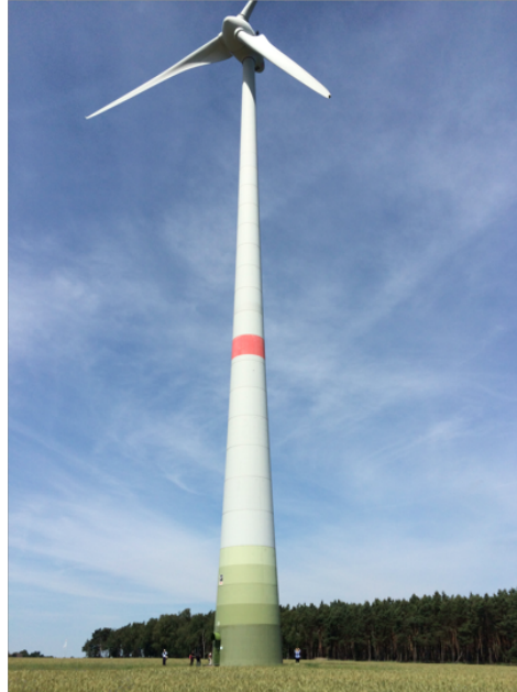
Figure 2. CREATE Participants enter the base of an Enercon turbine at the Feldheim wind farm.
