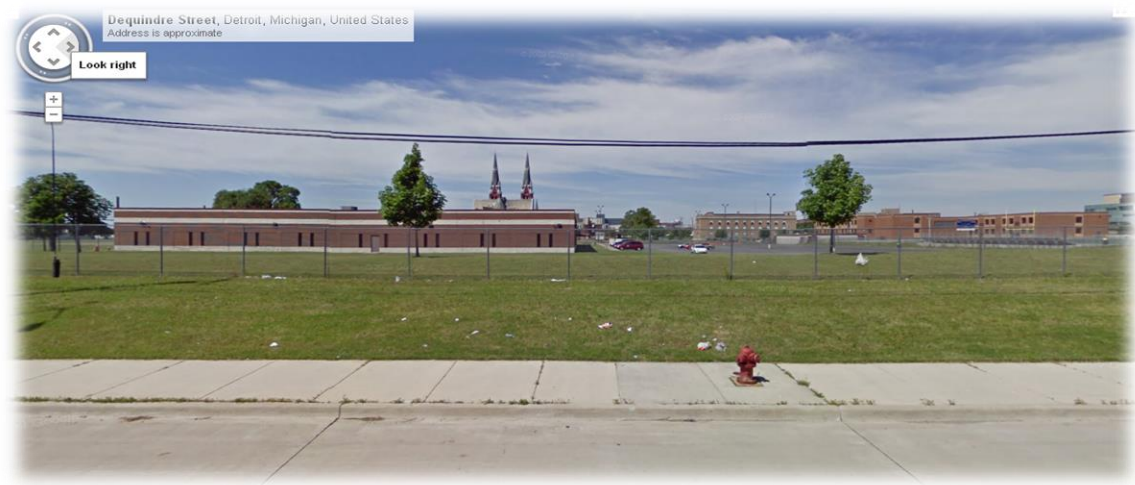
Figure 36. Dequindre facing west. This figure is taken from the same spot as Figure 35 but faces west with a view of the eastern side of PEC and the Family Services building to the right.
