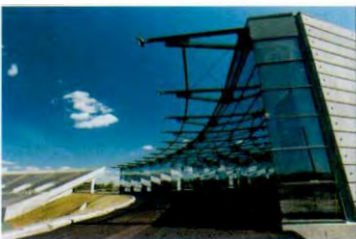
The new convocation center nears completion
