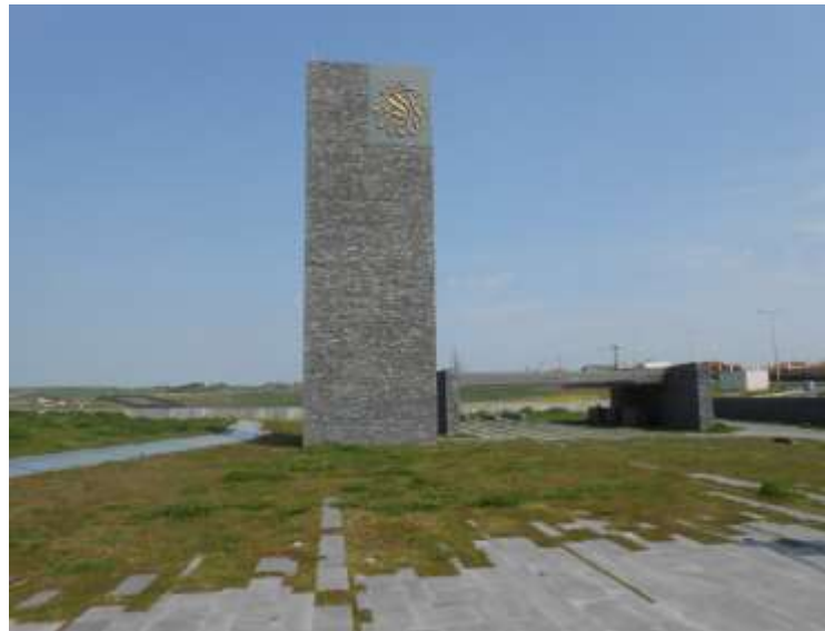
Figure 28. Sancaklar mosque minaret. (Pearson, 2014). Photo by: Thomas Mayer
