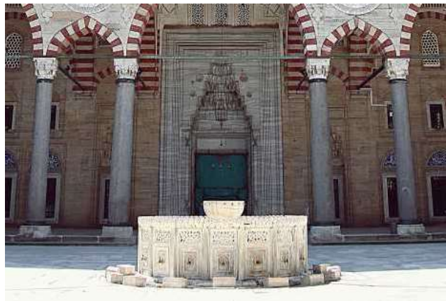
Figure 5. Selimiye mosque main entrance. (Okcu, 2014).
