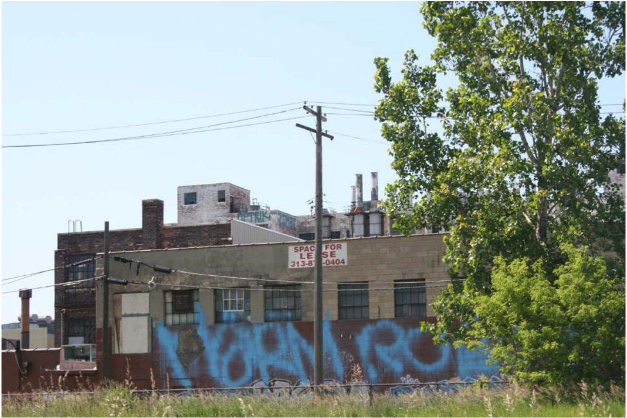
Figure 3.11. Building with graffiti in front of Fisher Body 21, Detroit, Michigan
