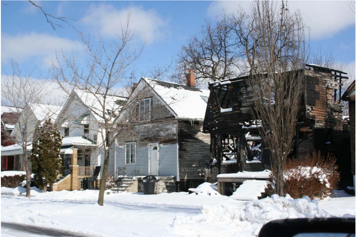
Figure 4.8 Abandoned home in Detroit (Catherine W. Barber)
