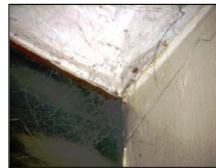
Figure 310 (right): Artwork is separation from the wall.
