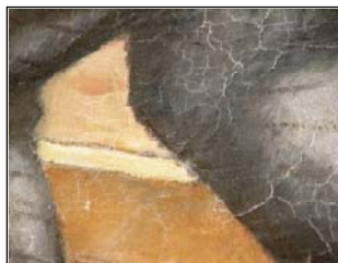
Figure 38: Deterioration of paint with noticeable crackling.
