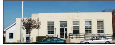
Figure 294: Rogers City, Michigan, post office.
