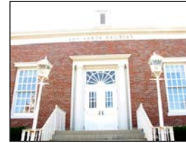
Figure 195: The original post office building; now owned by Ann Arbor Rail Road.
