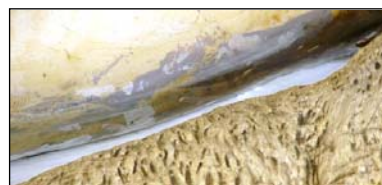
Figure 261: Visible spalling.
