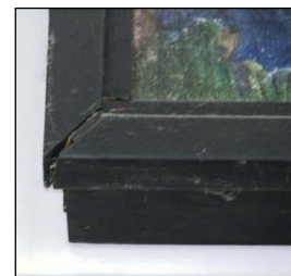
Figure 200 (right): The frame corners are separating. Perhaps the frame is covering the signature.
