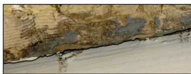
Figure 262: Visible spalling.
