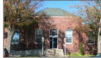
Figure 156: Frankfort, Michigan, post office.
