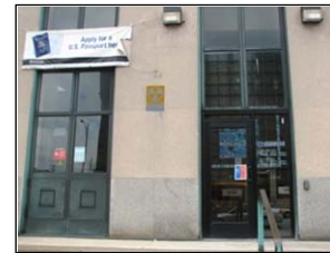
Figure 102: Detroit, Highland Park, Michigan post office.
