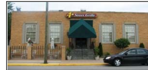
Figure 283: The former Rochester, Michigan post office where the artwork was originally installed.
