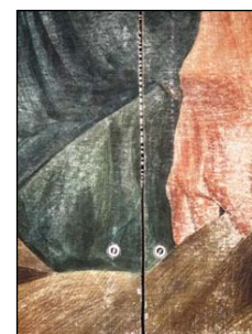
Figure 115: The mural was cut in half; bolts through the artwork attach it to the wall.
