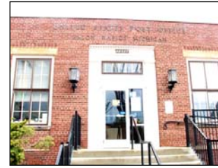
Figure 144: Eaton Rapids, Michigan, post office.
