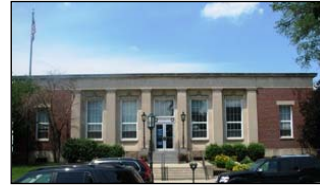
Figure 27: Birmingham, Michigan, post office.
