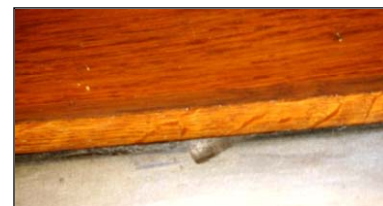
Figure 20: Frame separation and infestation.
