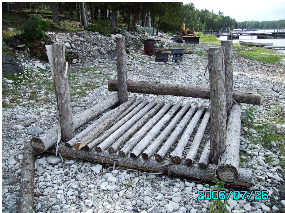
Figure 9. Dock Crib Being Constructed with the Floor In Place
