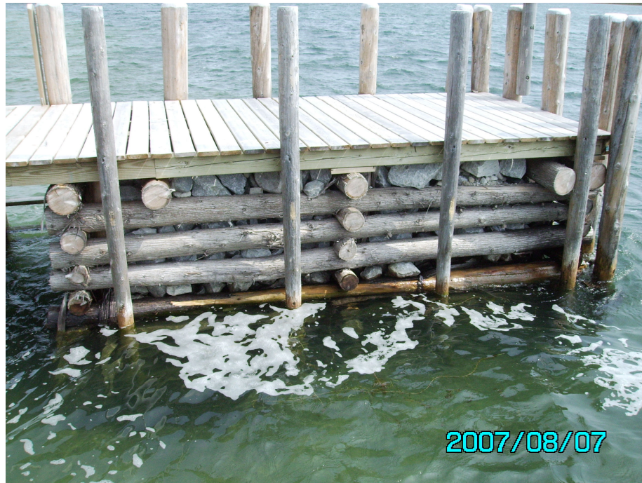
Figure 16. Dock End Pilings with Close Interval Spacing and Corner Clusters.
