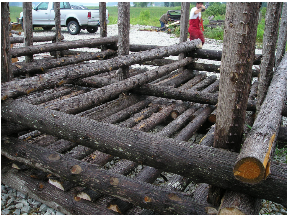
Figure 15. Oversized Crib Framework with Cross Bracing
