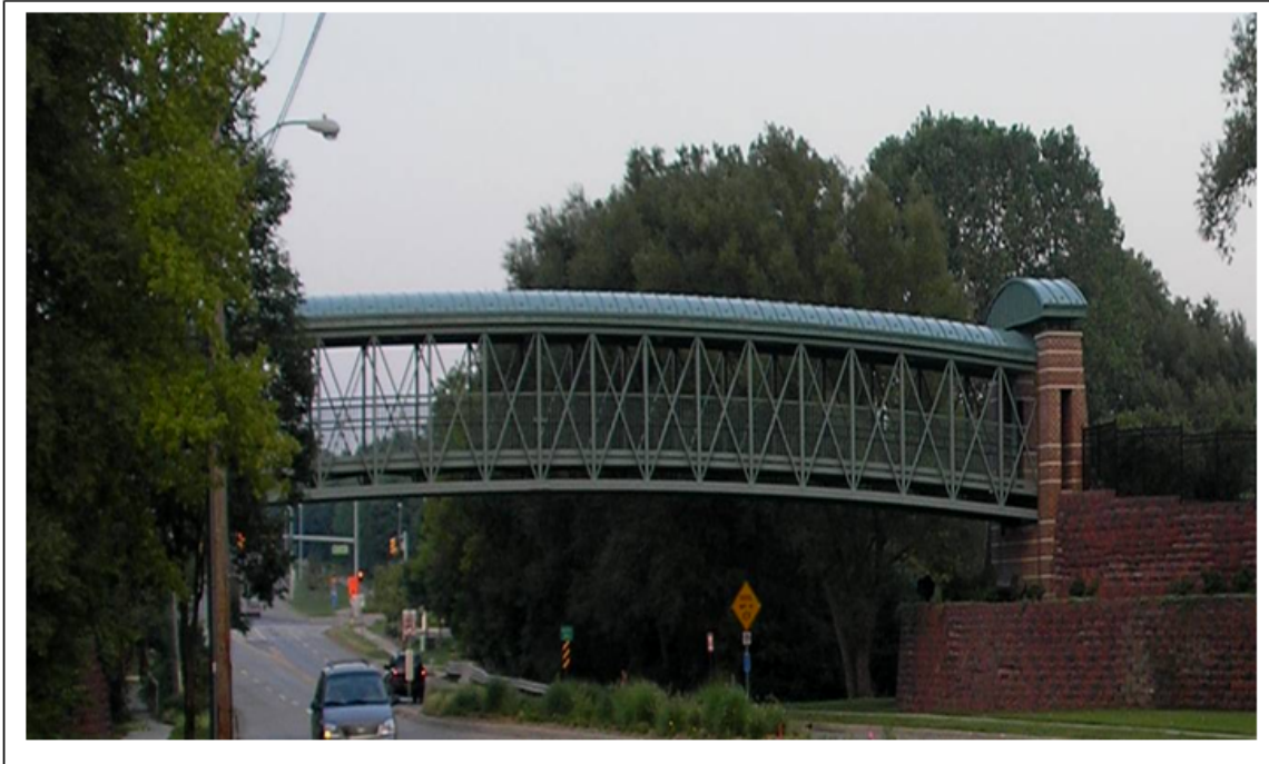
Figure 44: Pedestrian Walking Bridge on Milham Road
