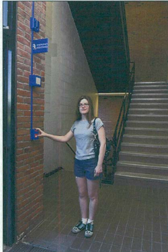
FEELING SAFE: Audrey Johnson demonstrates how accessible the alarm is at the emergency assistance station installed at Mark Jefferson this summer. Another station is located in Strong Hall. Photo by Randy Mascharka
