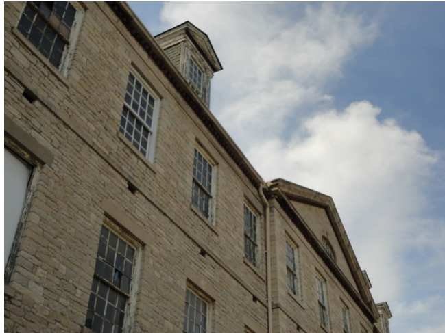
Exterior shot of Fort Wayne
