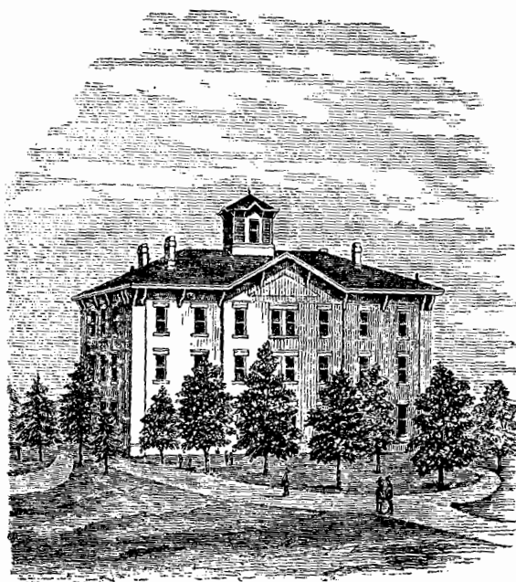
Building Restored After the Fire, 1860.
