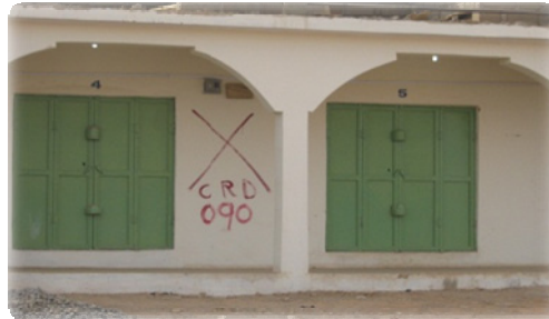
Figure 1. Marking the Structures with Red “X”
