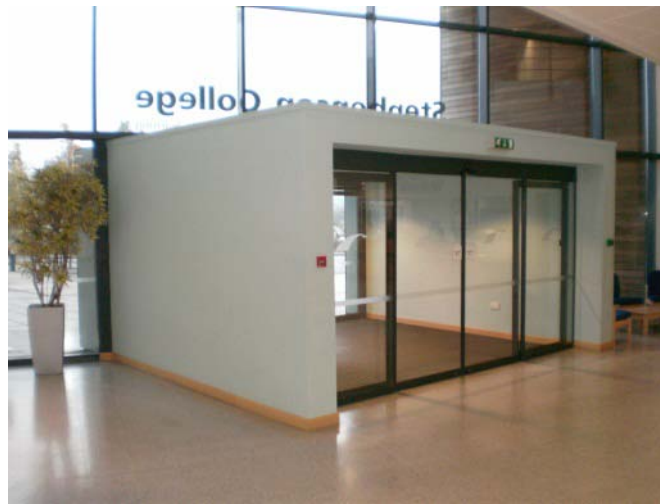
Figure 1. Image of the Front Entrance “Vestibule”
