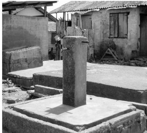
Figure 4. Pipe Borne Water in Lobe Estate: A Legacy of Pamol Plantation
