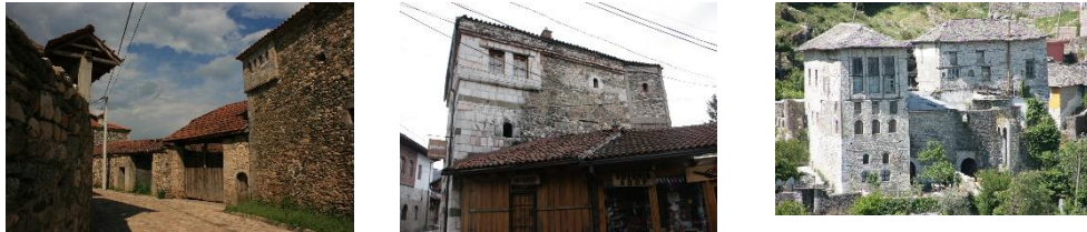
Fig. 2. Traditional tower houses combined to a fortress-like compound in the countryside (Dranoc - left ); urban tower house in the middle of the market area (Gjakova - center ); freestanding, comfortable tower residences forming a neighborhood (Gjirokaster - right ); all photographs by Jaeger-Klein
