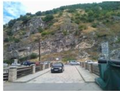
Fig. 4. Bridge for vehicle access.
