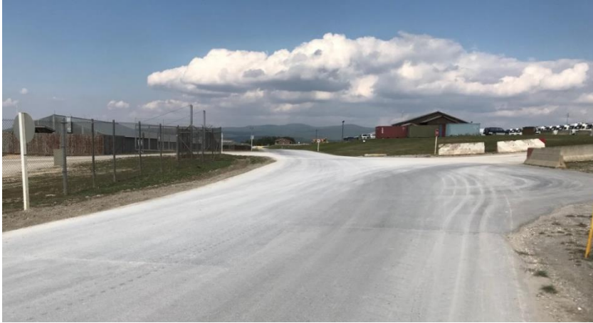
Fig 4: Replaced concrete with asphalt pavement at 2nd road intersection on Bondsteel
