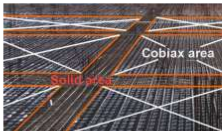
Fig 1 The appearance of cobiax slab surface and the solid area.
