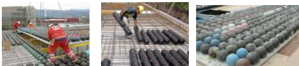
Fig 4 Application of prefabricated slabs in site
