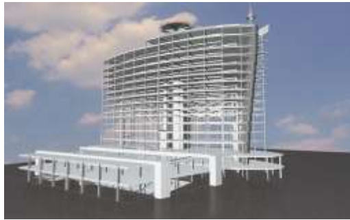
Fig 9 A view of building construction
