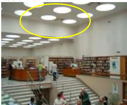
Fig. 27. Interior of conical skylights
