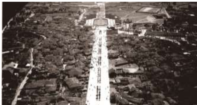
Fig. 11. Aerial photo of Skanderbeg square, in 1936 ( Archive of IGM, Firenze)
