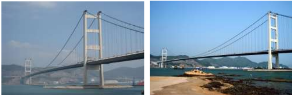
Foto 1 Tsing Ma Bridge : http://www.patnotebook.com/tsing-ma-bridge-photos-and-how-to-get
