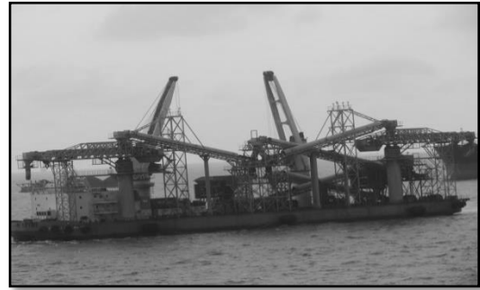
Gambar 2. Floating Crane Mutiara Jawa 1
