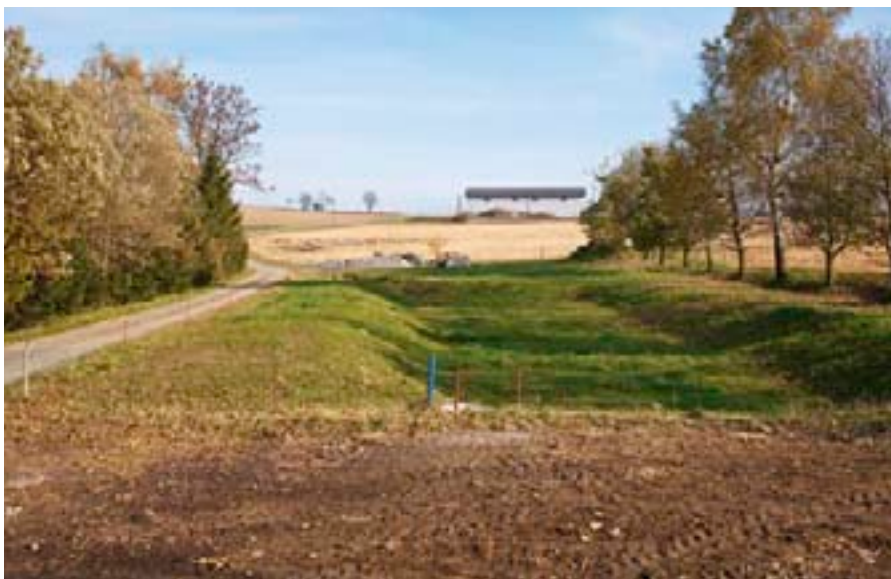
Completed flood-water storage pond – catchment area A 2
