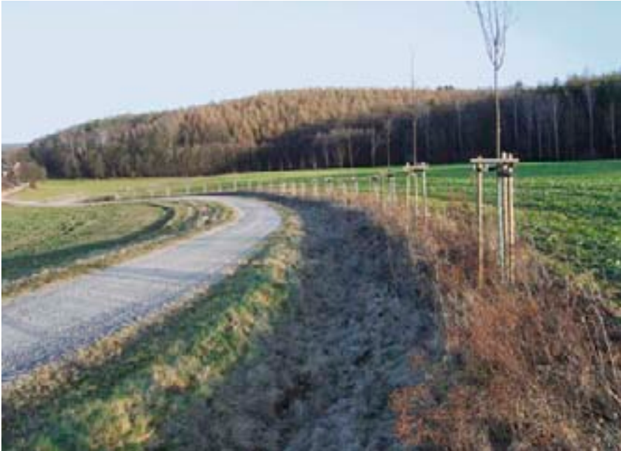
Bräuneck Weg after completion; photo: Dr. Gunter Möbius
