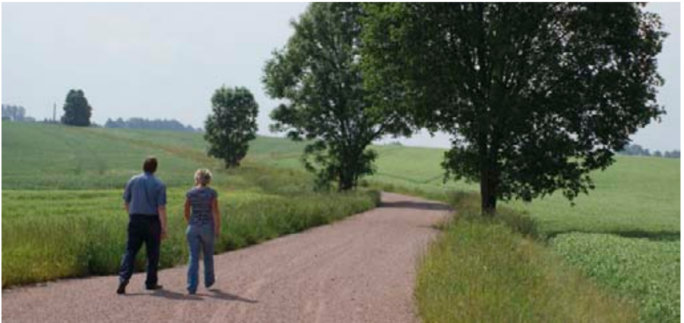
"Stichweg" after the expansion
