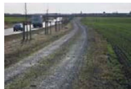
Creating a new access road parallel to the local by-pass; photo: S 177 OU Radeberg/GroBerkmannsdorf Community of Participants
