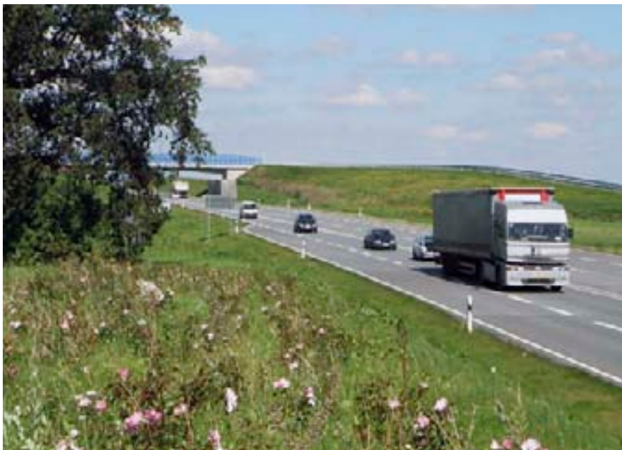
The opening to traffic on the S 177 subsection, local by-pass Radeberg–Großberkmannsdorf in December 2008
