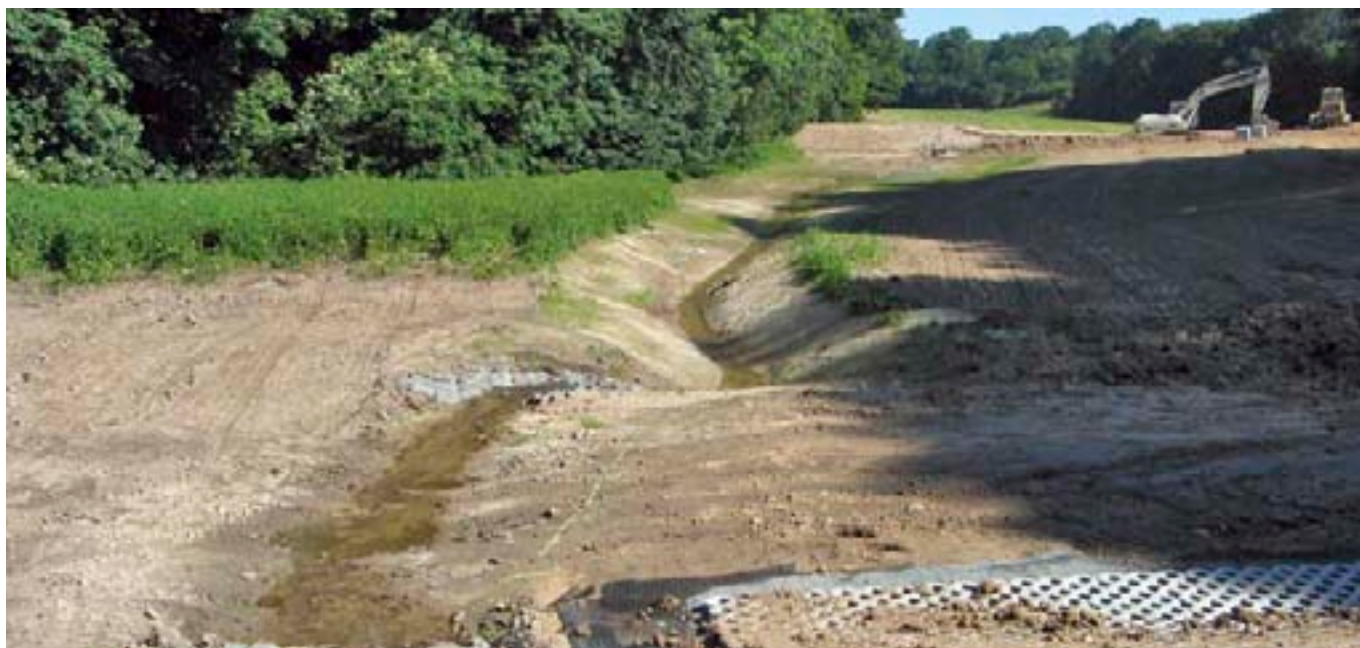
Near-natural reshaping of the Ziegenbach ground; photo: Zschadraß (Hochwasser-) Muldedörfer Community of Participants
