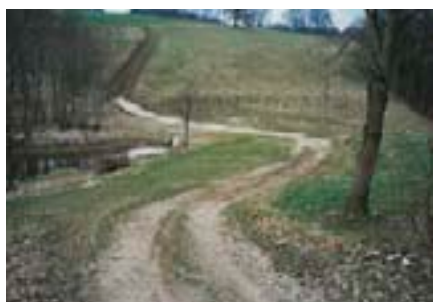
Unspoilt pond with emergency overflow; photo: Zschadraß (Hochwasser-) Muldedörfer Community of Participants
