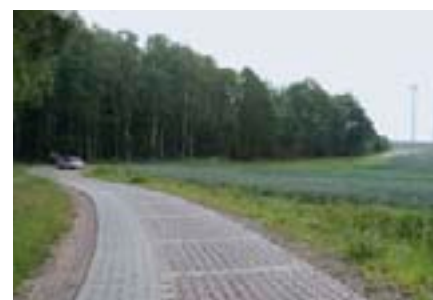
"Südlicher Querweg" – section with a paved surface of concrete blocks
