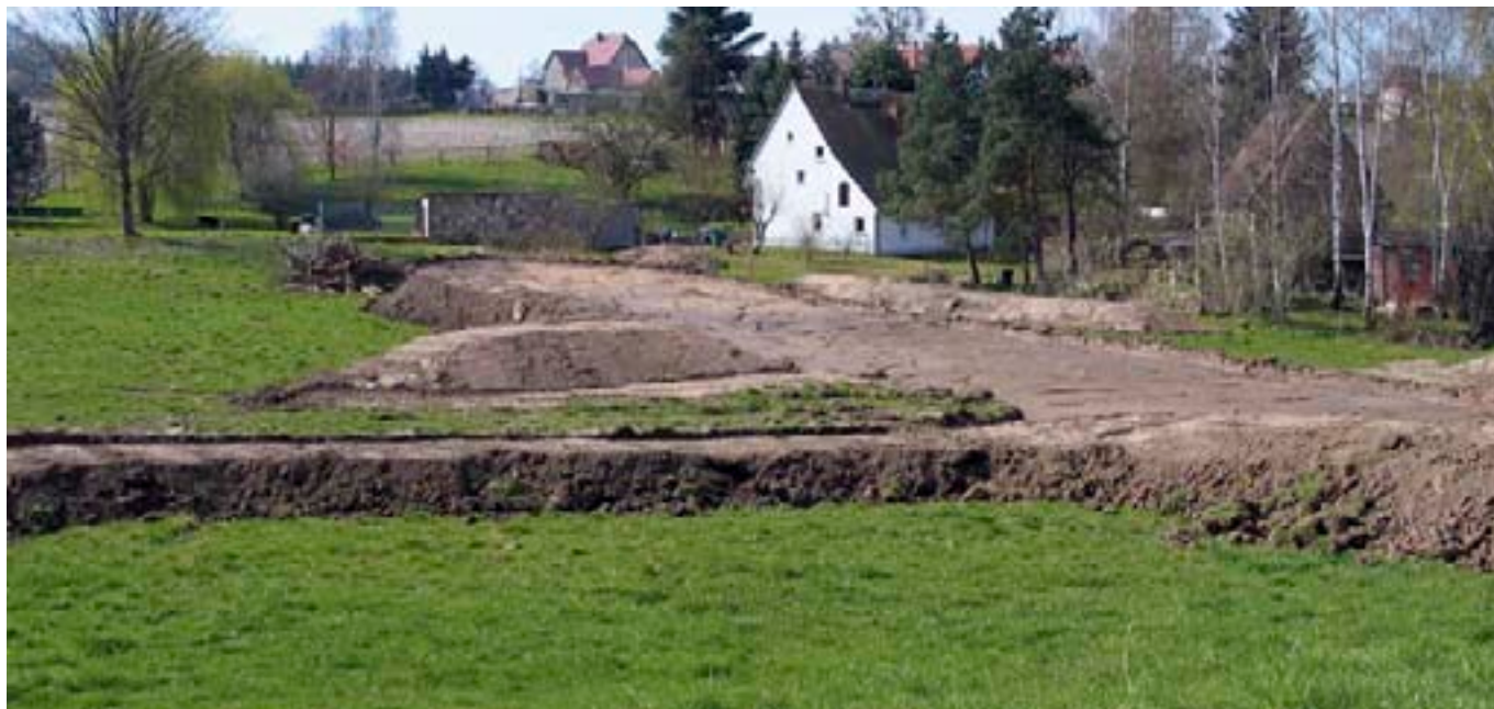
System of flood protection embankments above the locale of Podelwitz; photo: Zschadraß (Hochwasser-) Muldedörfer Community of Participants
