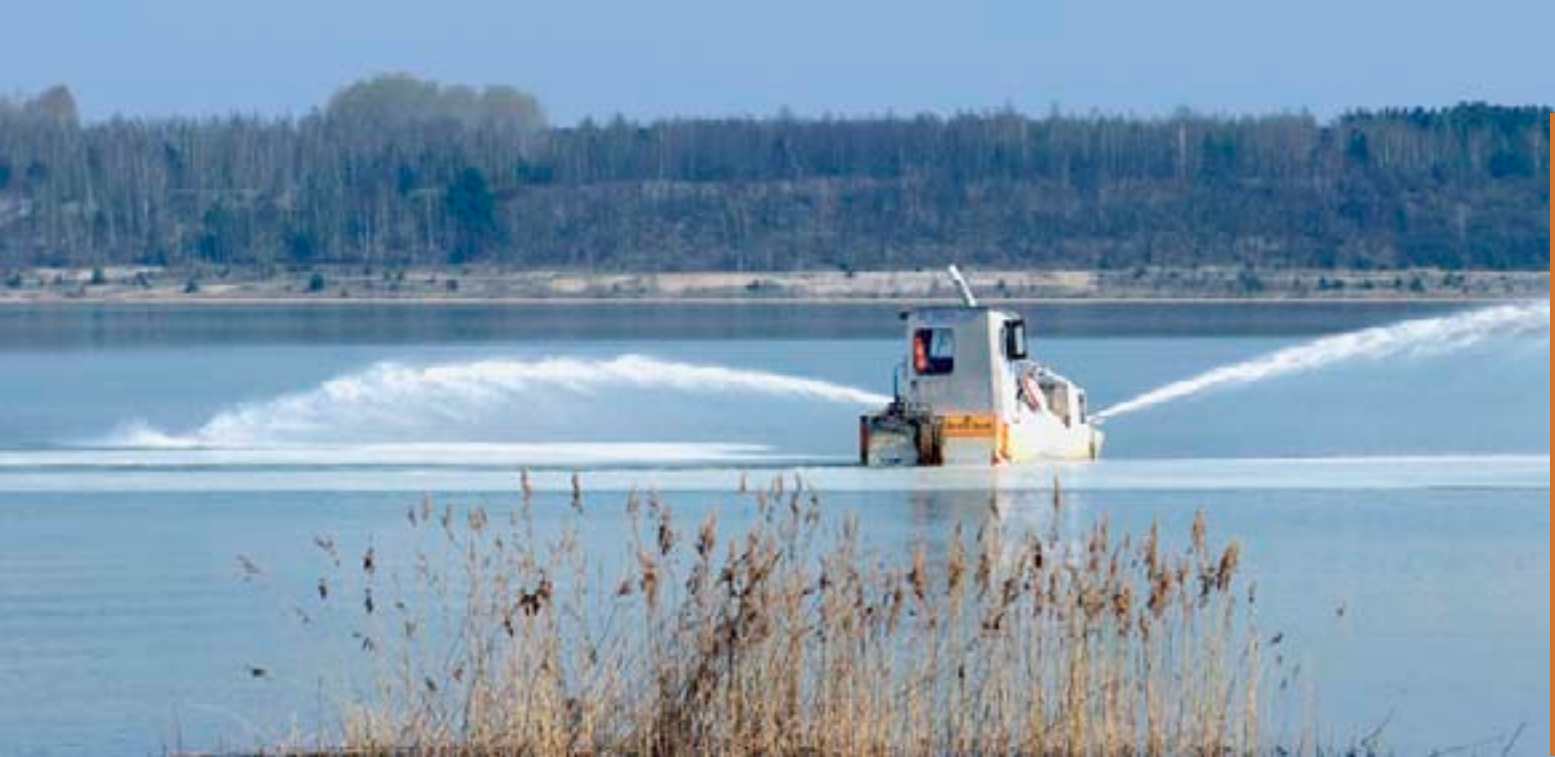
Remediation ship on Haselbacher See; photo: LMBV
