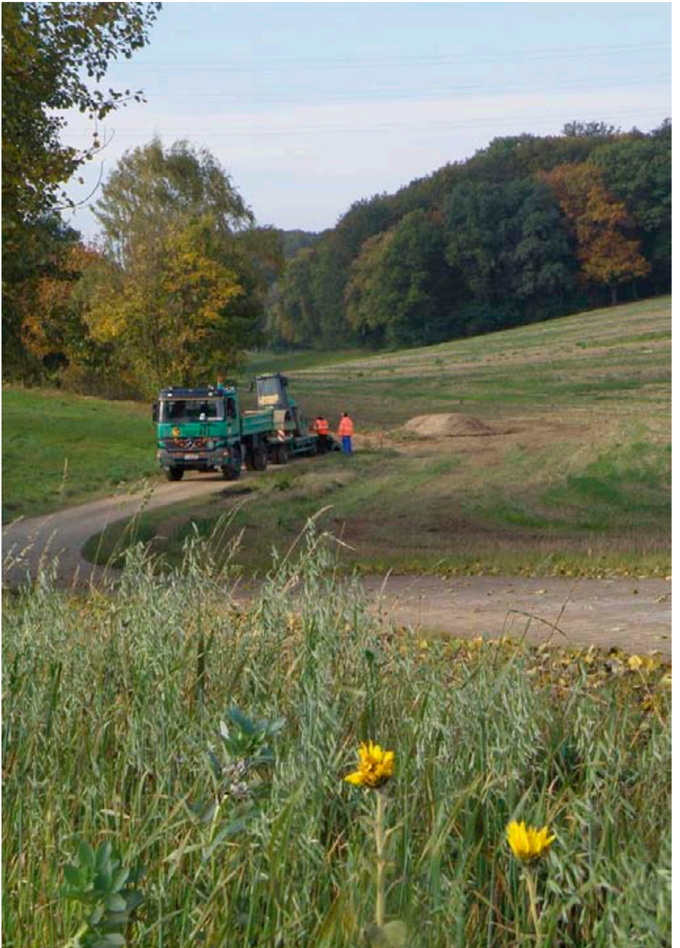
Construction of a rural on Schönberg farmland
