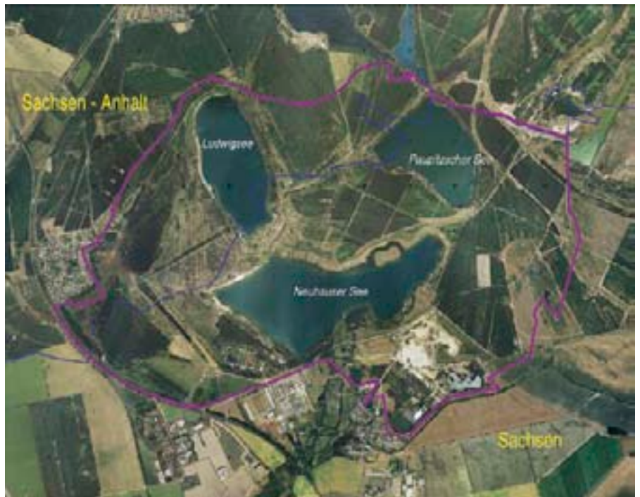
Overview map of the land consolidation area (red boundary) showing the state border (identified in blue); Lake Ludwig (top left), Lake Paupitzsch (top right), Lake Neuhaus (bottom); photo: LMBV
