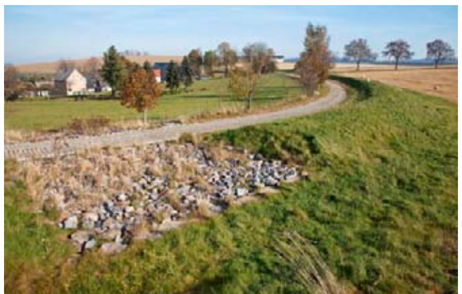
Completed flood control dam with spillway and farm road – catchment area A1. The locale to be protected is seen in the background.
