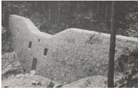
Slot barrier, 19 th Century (Lünitzbach, Kärnten-Austria) Slit barrier, 19 th Century (Reißgraben, Kärnten-Austria)
