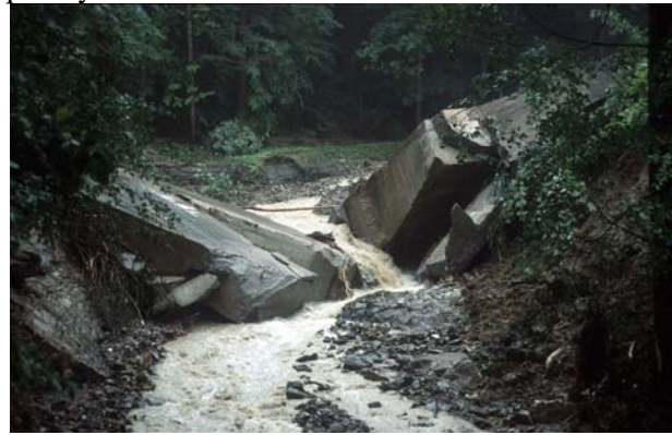
Scouring and/or inadequate design
