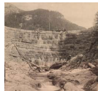
Sediment control barriers
