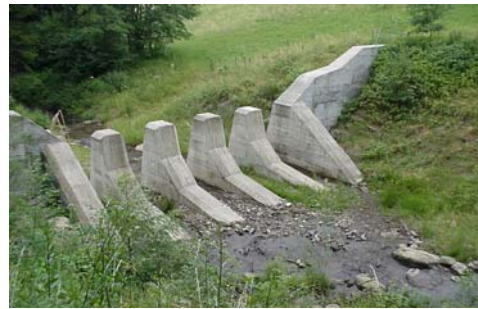
Sectional beam barrier (Niedernsiller Mühlbach, Salzburg-Austria) Sectional barrier with fins (Gemmersdorferbach, Kärnten-Austria)
