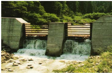
Sectional beam barrier (Niedernsiller Mühlbach, Salzburg-Austria) Sectional barrier with fins (Gemmersdorferbach, Kärnten-Austria)
