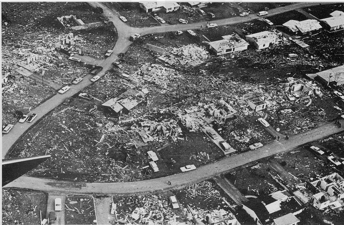
FIGURE 24. Severe damage in the residential section of Crystal Lake, Illinois that occurred at 3:27 p.m. CST on April 11; picture was taken on April 12. (For exact location, refer to Aerial Survey Map No. 4)
