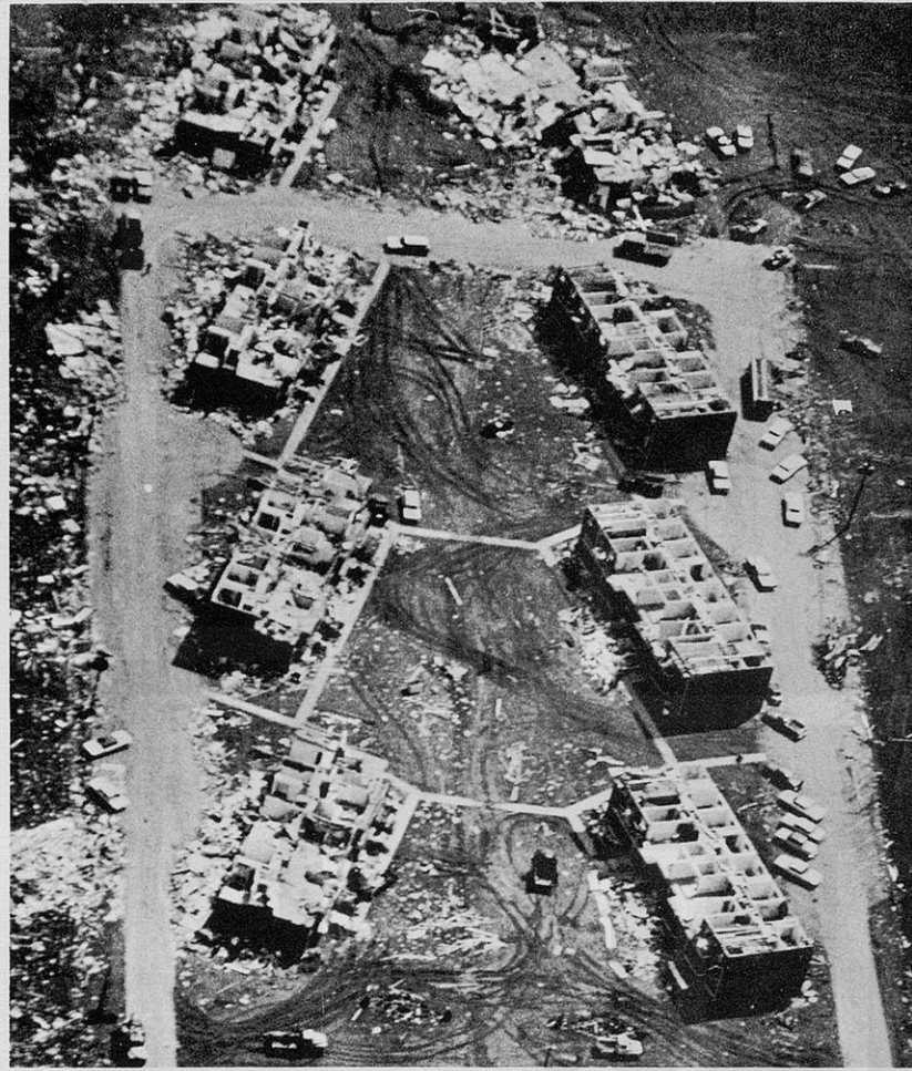
FIGURE 37. Eight brick apartment buildings south of Kokomo, Indiana in various states of destruction ranging from loss of roofs to collapse of walls. Destruction occurred at 6:43 p.m. CST, April 11; picture was taken April 16. (For exact location, refer to Aerial Survey Map No. 13)
