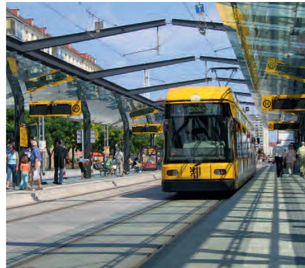
The central public transport interchange "Dresdner Postplatz"
