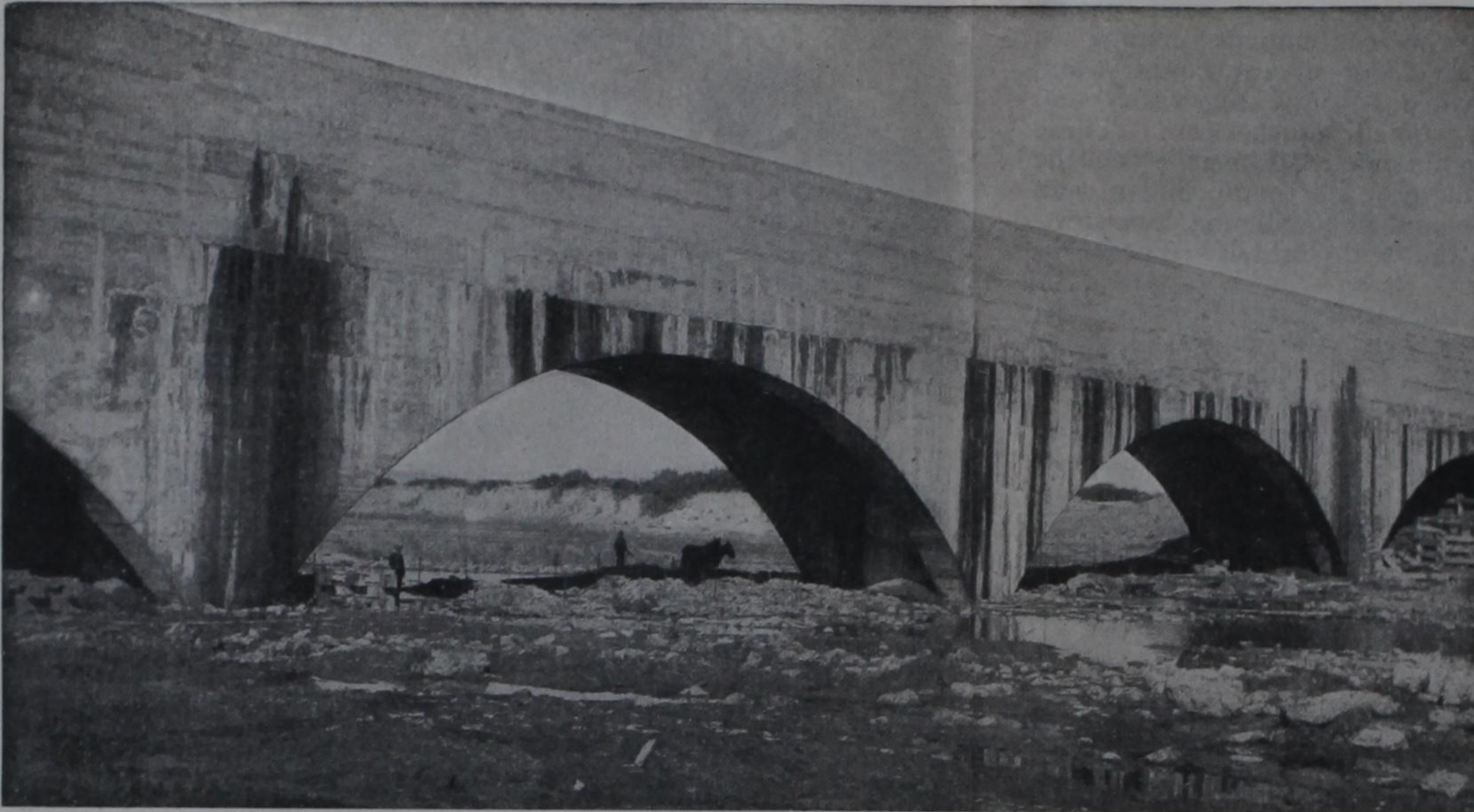
Aqueduct that Spans the Pecos River, near Carlsbad, New Mexico.
