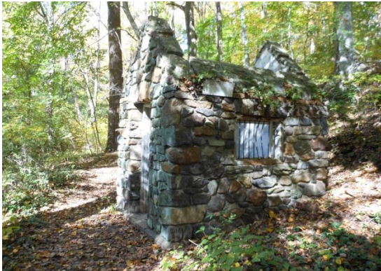
Stone structures in Houston Park
