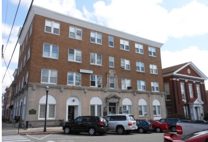
County Court Apartments Site of former regional FBI office involved in 1971 burglary (Second floor, left side) Photo: Walt Cressler, 2013
