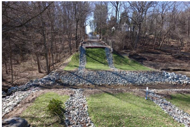
The former dam in 2018
