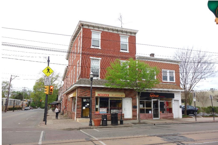
Nooddi the Noodle Bar – former building for Carey & Brother Plumbing Photo: Walt Cressler, 2018
