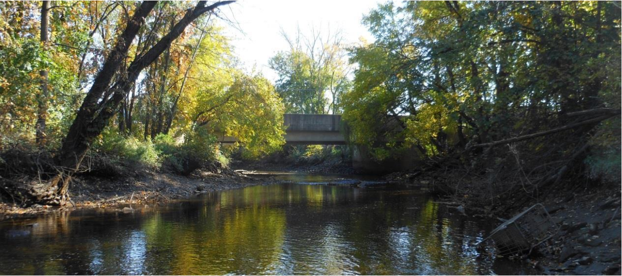
Ridley Creek flowing towards the Chester Pike bridge
