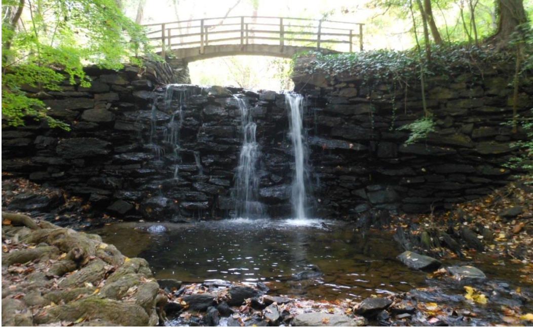
Vernon Run below the dam, Rose Valley
