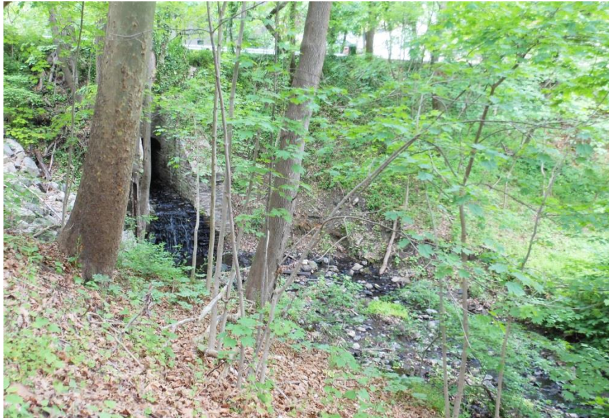
Outfall of small tributary that flows from one park to the other Photo: Walt Cressler, 2012
