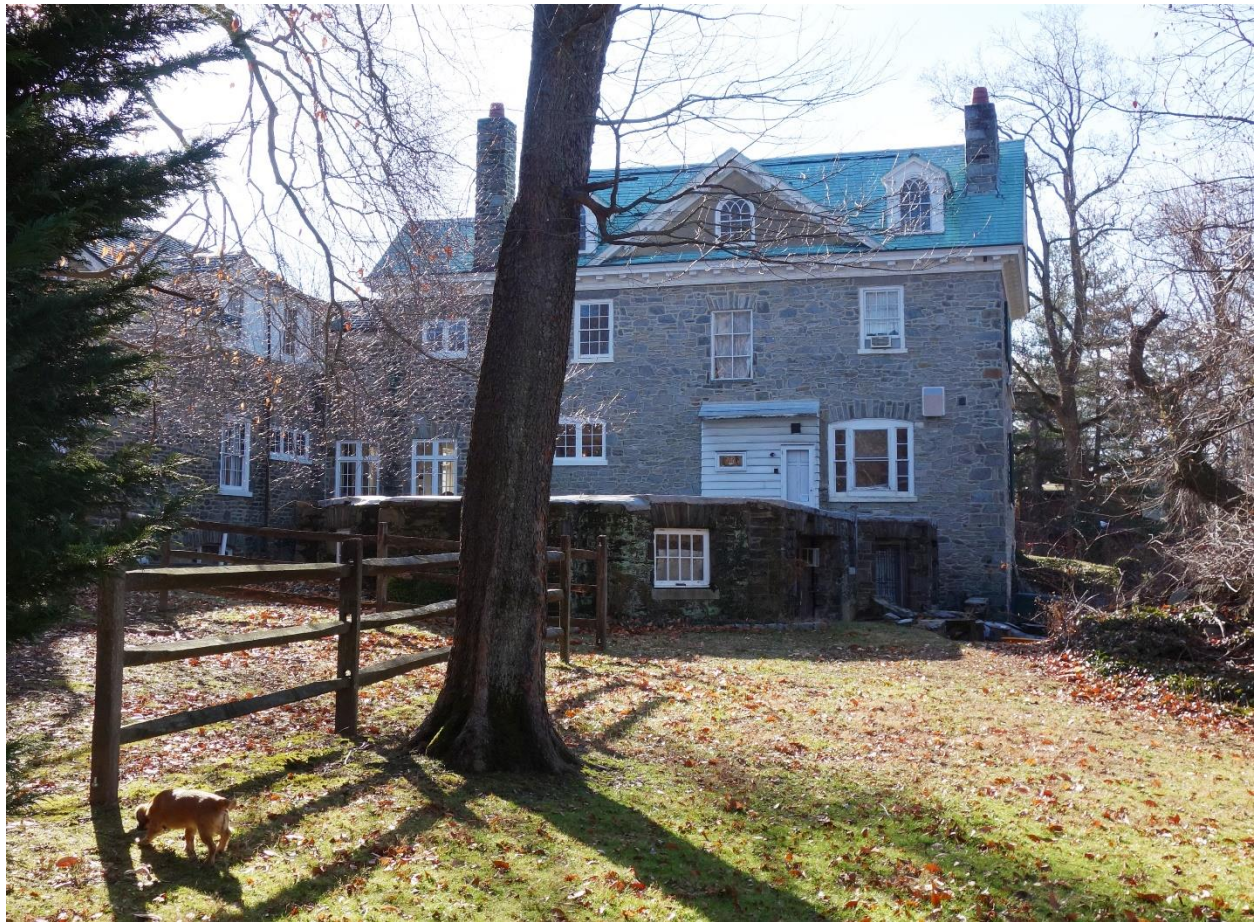
Rear of Lapidea Mansion, showing remnants of the Sproul additions.
