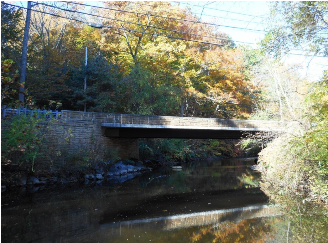
Ridley Creek under the Knowlton Road bridge
