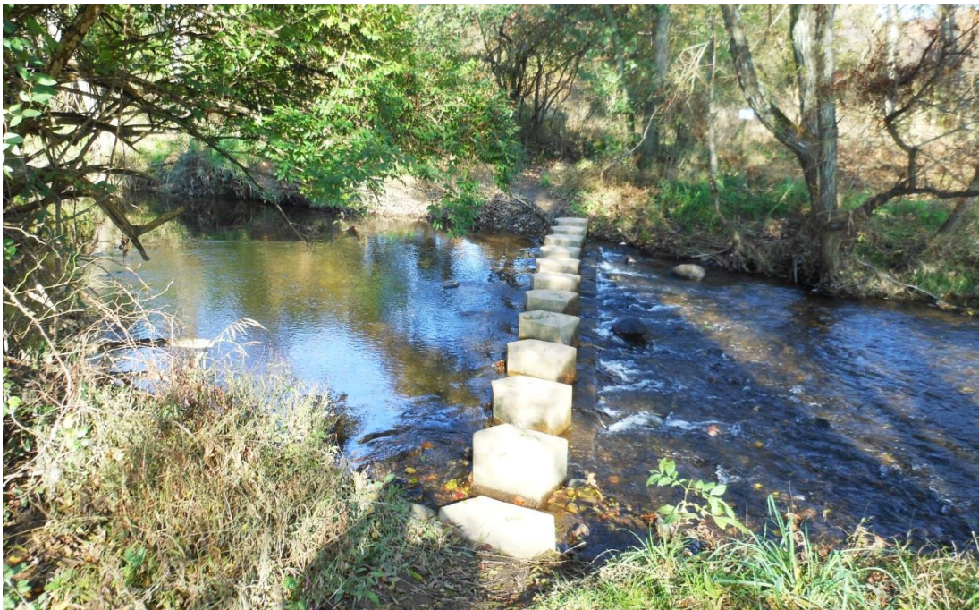
Step bridge across the Ridley, Ashbridge Preserve
