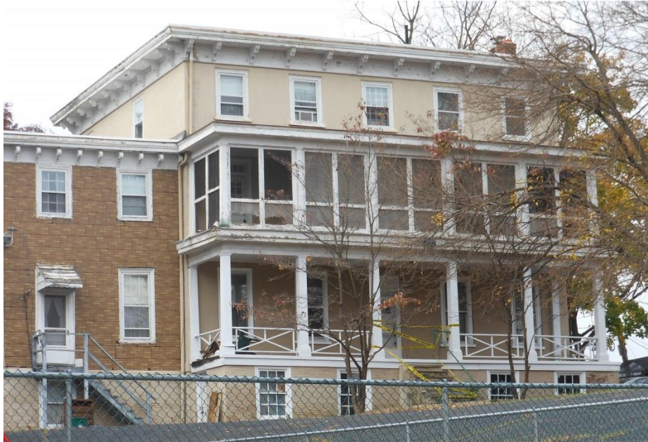
Another view of the former Gayley Classical Institute Photo: Walt Cressler, 2012
