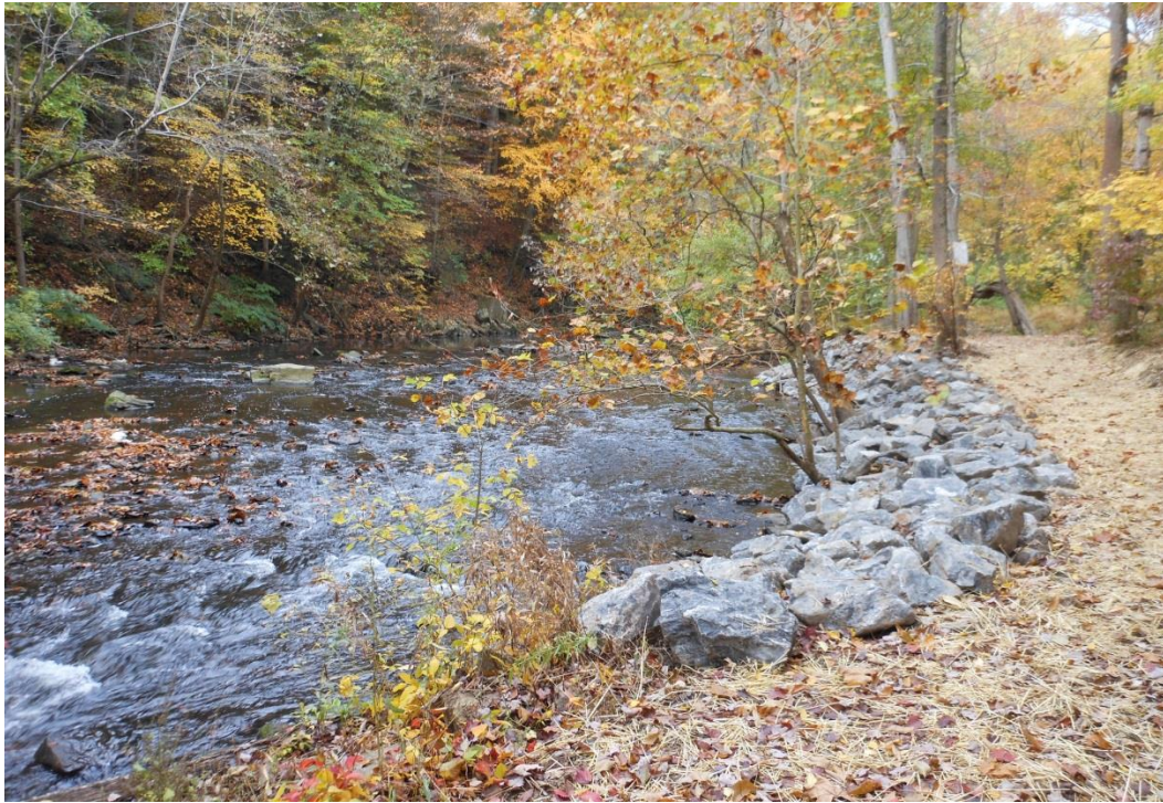
Stream bank restoration project
