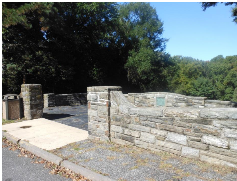
Entrance plaza to Glen Providence Park, State Street, Media Photo: Walt Cressler, 2012
