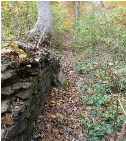
Remains of the millrace and millrace wall
