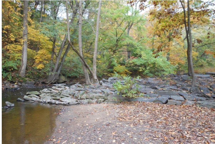
Remains of the dam
