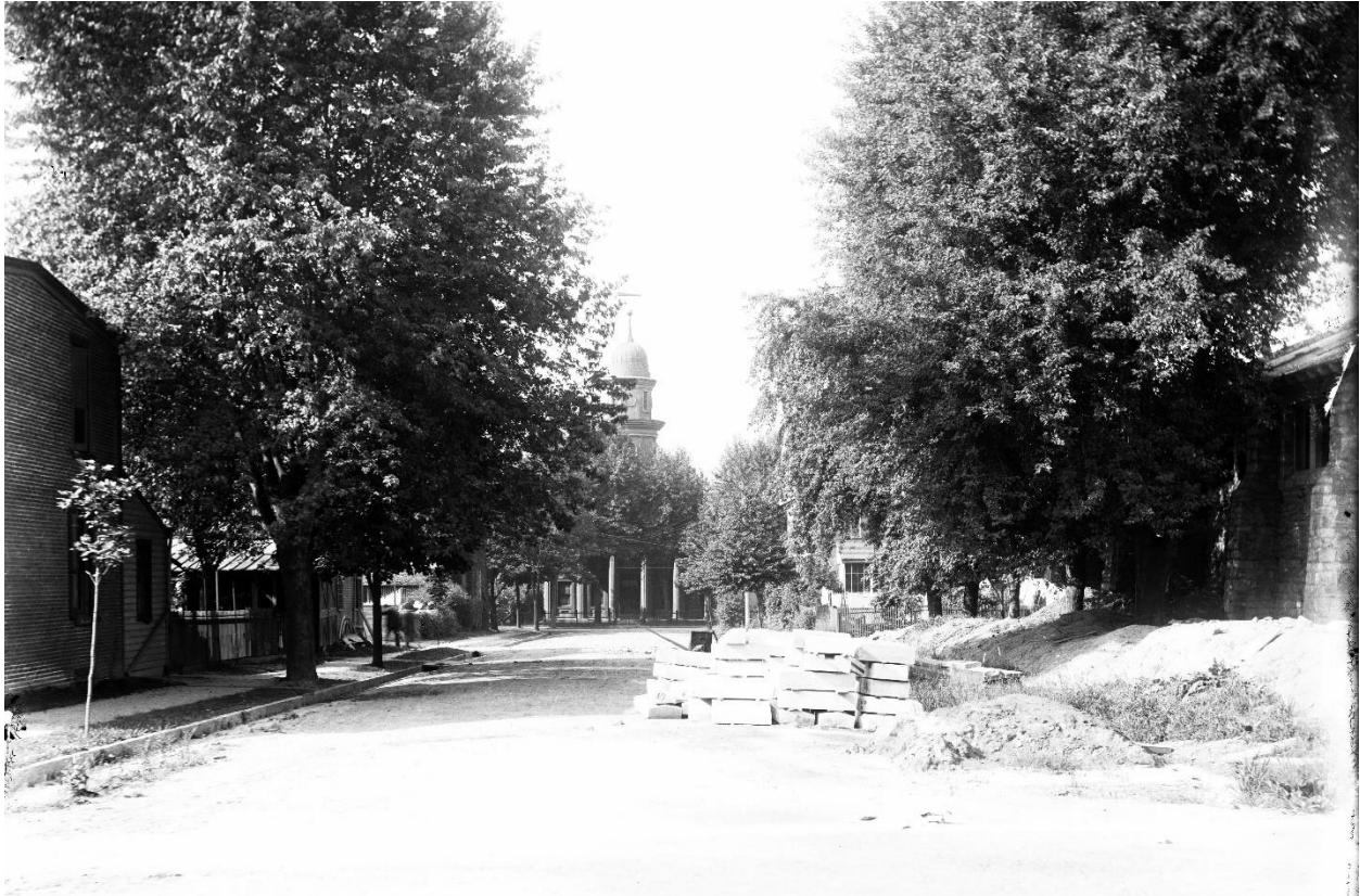
Church Street scene during the Armory construction, 1908 Photo: Stephen H. Appleton – Media Historic Archives
