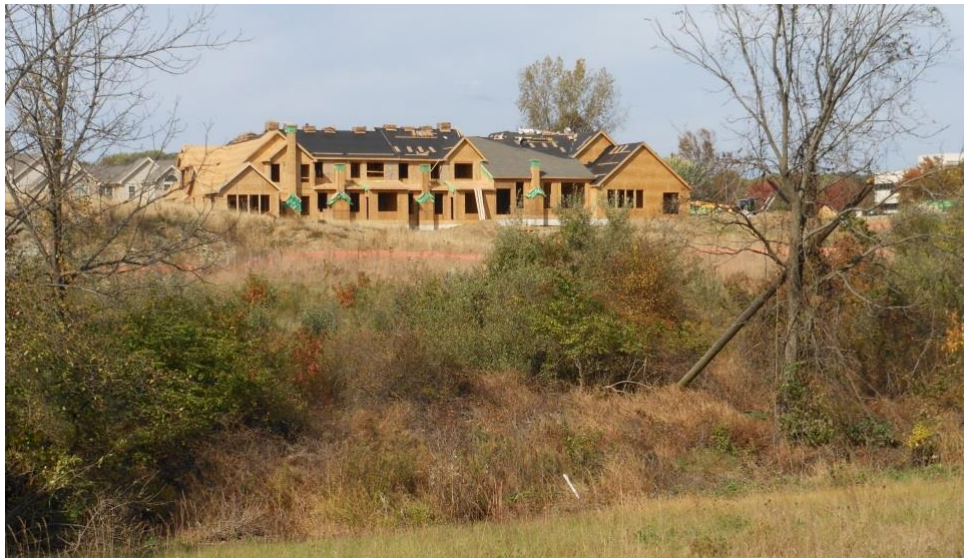
The construction of Applebrook Meadows subdivision Photo: Walt Cressler, 2012
