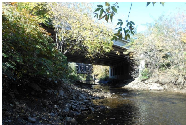
Ridley Creek under the Conrail and I-95 bridges Photo: Walt Cressler, 2012
