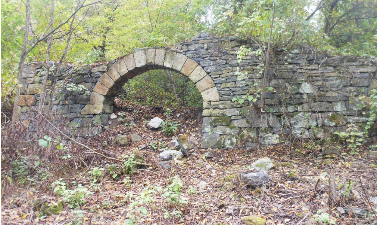
Ruin of the South Farm barn
