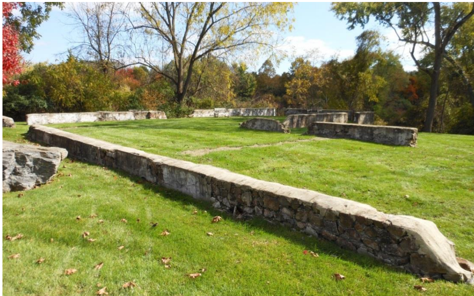
Foundation of George Smedley's barn, the oldest in Pennsylvania (1697)
