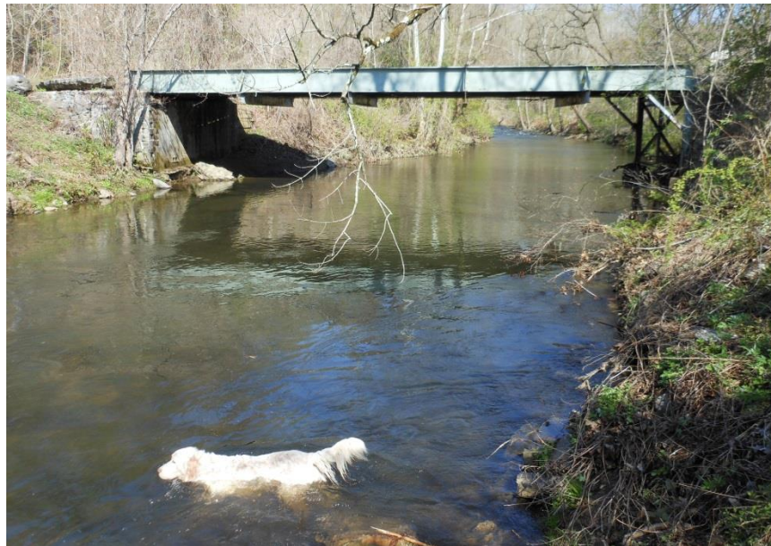
Ridley Creek under the Sackville bridge Photo: Walt Cressler, 2014
