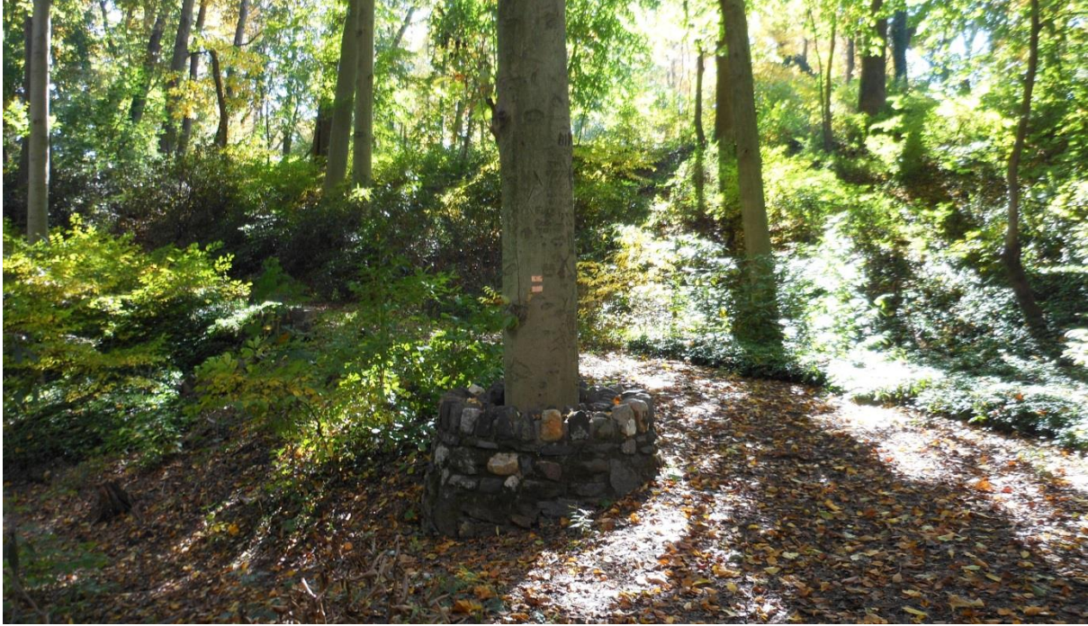
Circular wall around a beech tree, Houston Park
