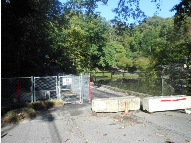
Broomalls Dam (condemned), Third Street, Media Photo: Walt Cressler, 2012
