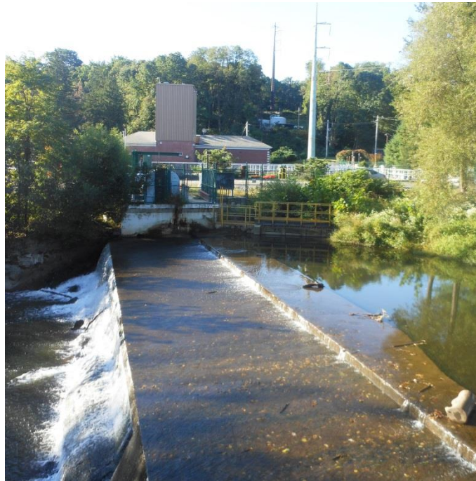
The dam at the Media Water Works Photo: Walt Cressler, 2012
