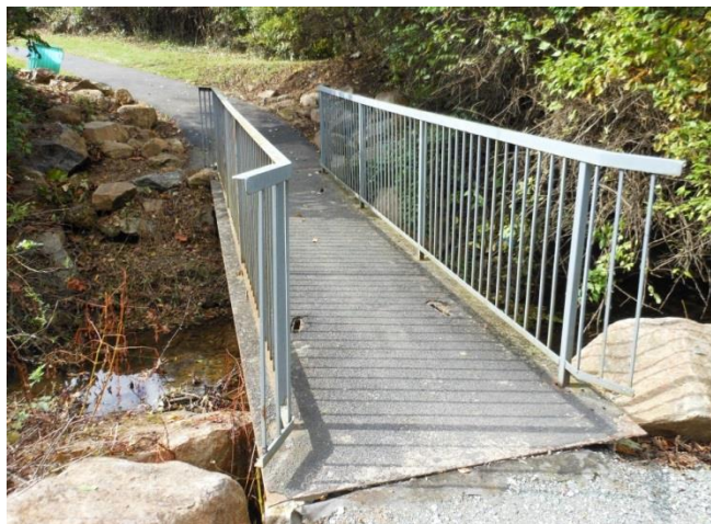
Foot bridge over George Smedley Run at the Hunters Run Condominiums
