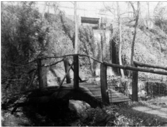
Broomalls Dam, bridge over run
