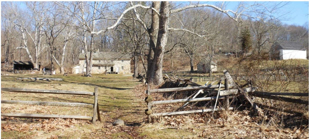
Colonial Pennsylvania Plantation, Ridley Creek State Park
