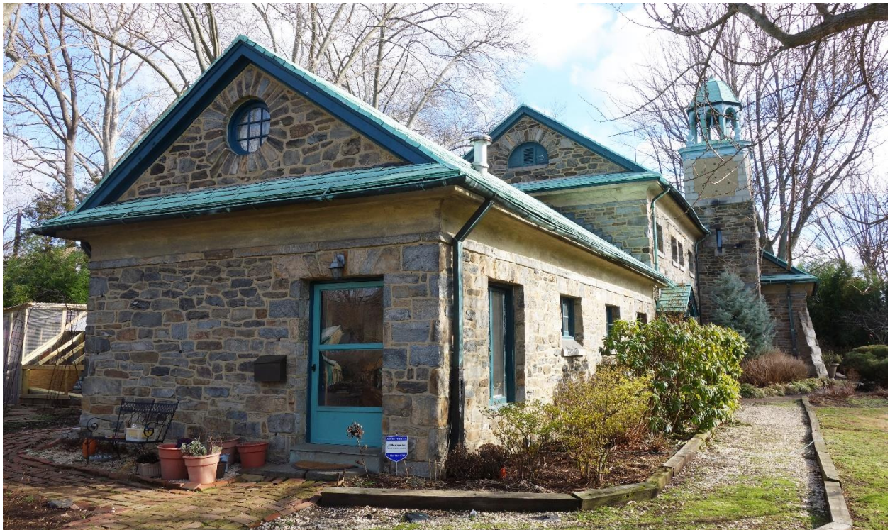
Two views of the Sproul stable/garage
