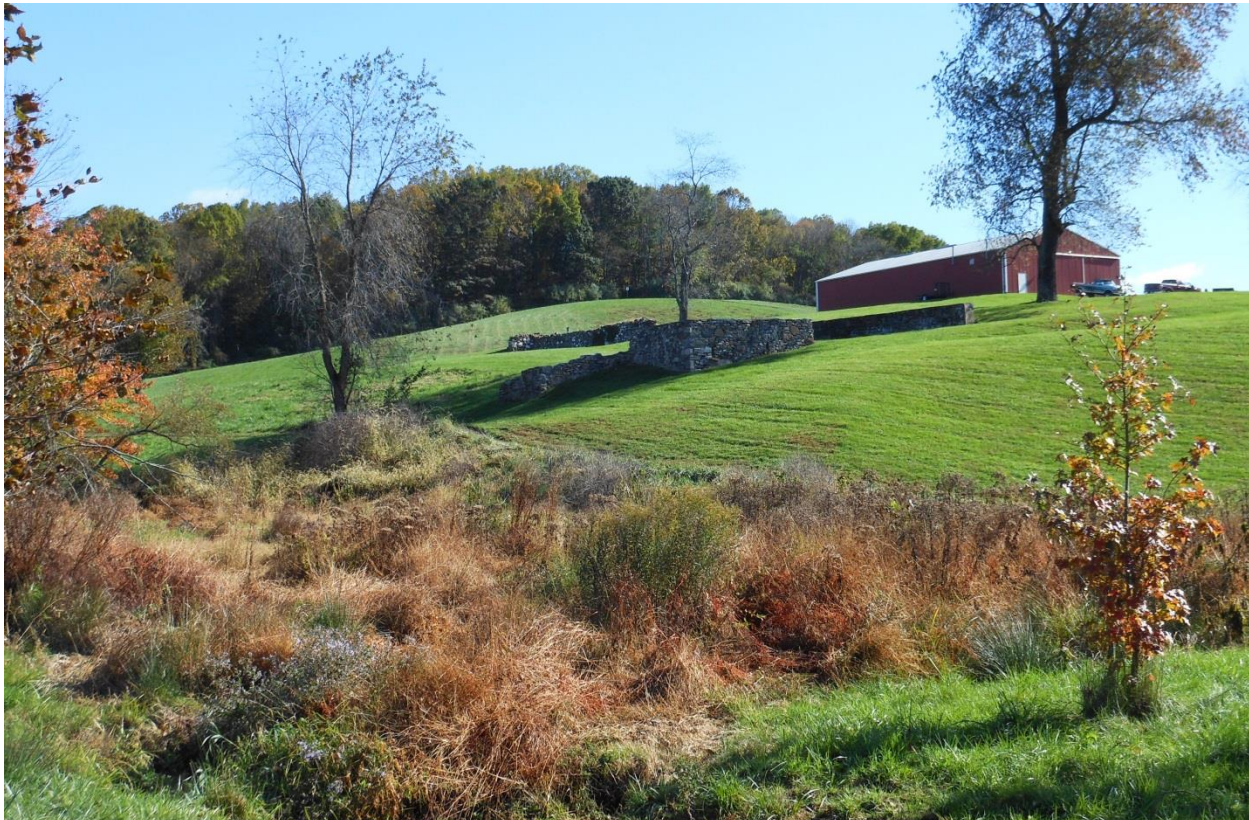
Delchester Run flowing below foundation of Garrett barn and Willistown Township utility shed Photo: Walt Cressler, 2012
