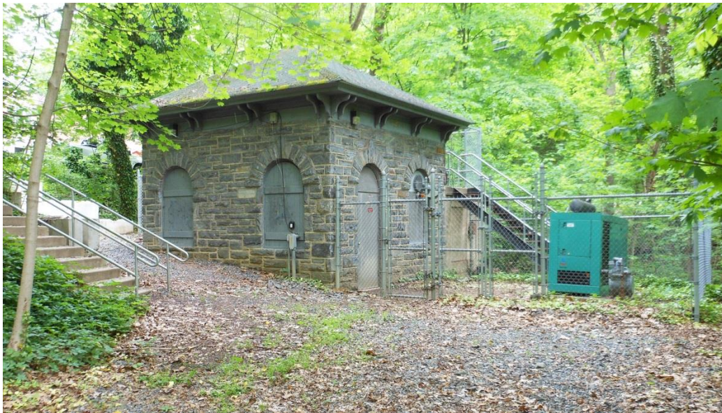
Sewage pump house, G.D. Houtman Park
