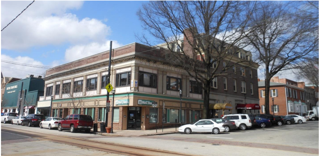
M & T Bank and Plymouth Apartments Former Media Title & Trust Building attached to the former Charter House Hotel Photo: Walt Cressler, 2013
