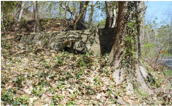
Remains of industrial operations, Middle Bank
