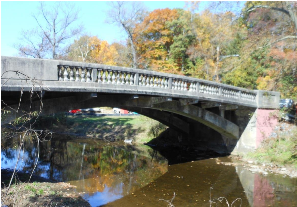
Bridge across Ridley Creek, Chester Park
