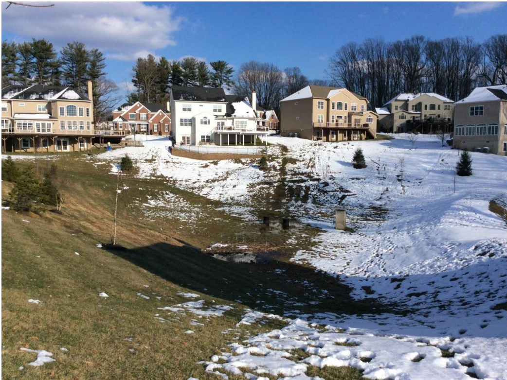
Stormwater basin in the Woodlands at Ridley Creek Photo: Walt Cressler, 2018
