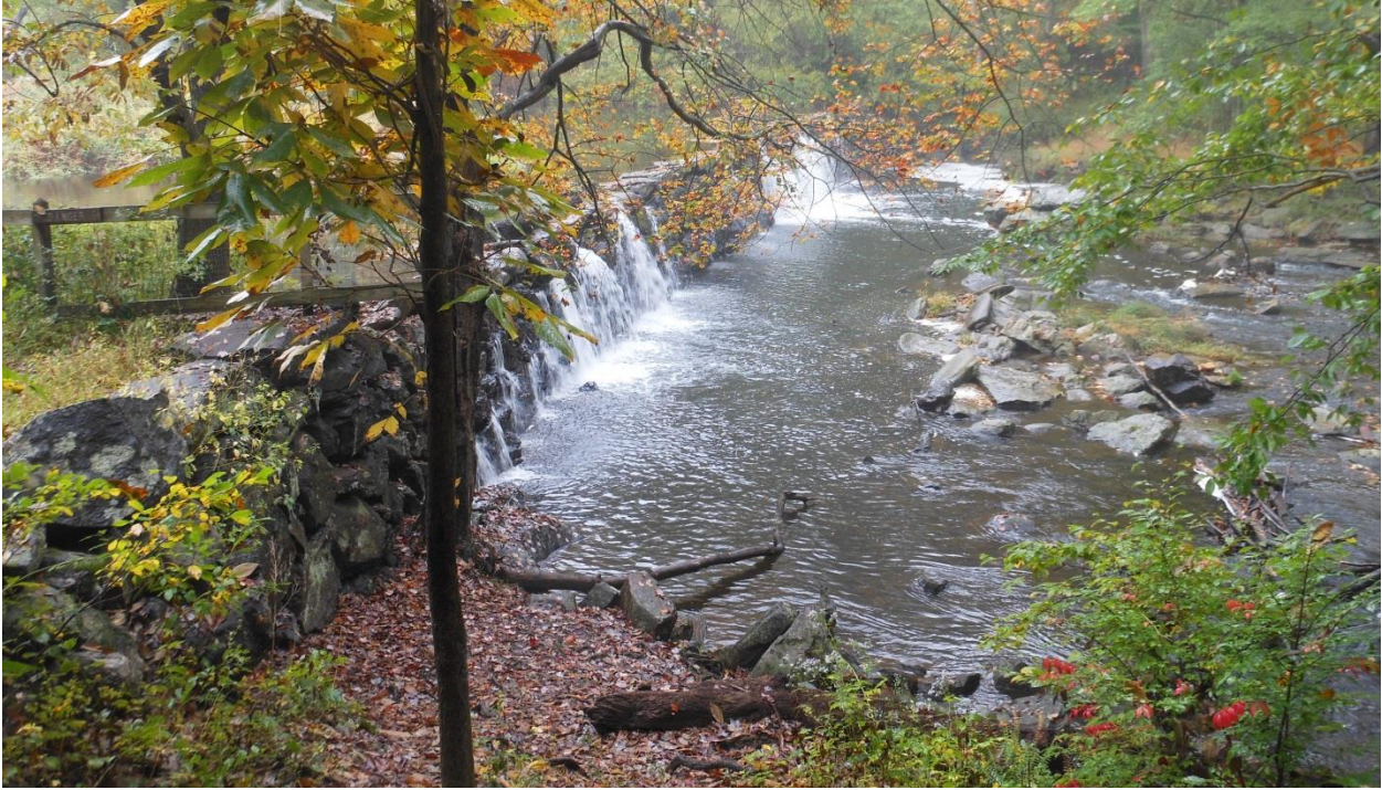
Sycamore Mills dam, Ridley Creek State Park
