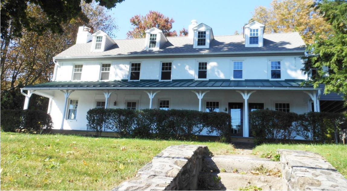
Briggs Farmhouse, newly restored
