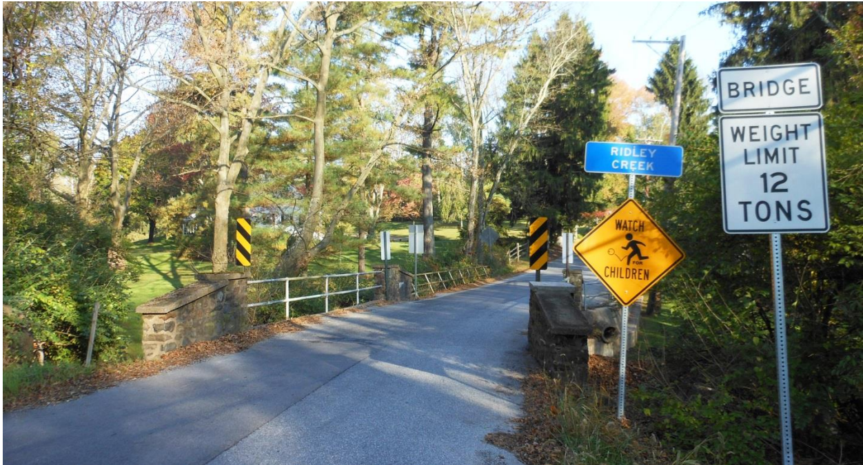
The bridge over Ridley Creek at Dutton Mill Road
