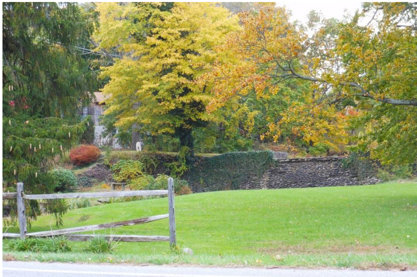
Hershey's Mill dam from Greenhill Road
