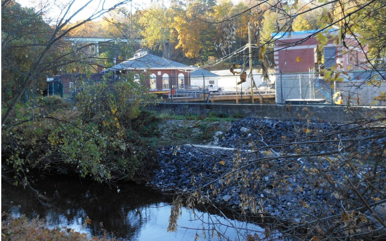
Media Water Works from Ridley Creek with Media-Elwyn Commuter Rail trestle in background Photo: Walt Cressler, 2012
