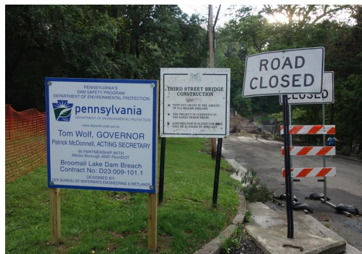
Signage at the Third Street breach
