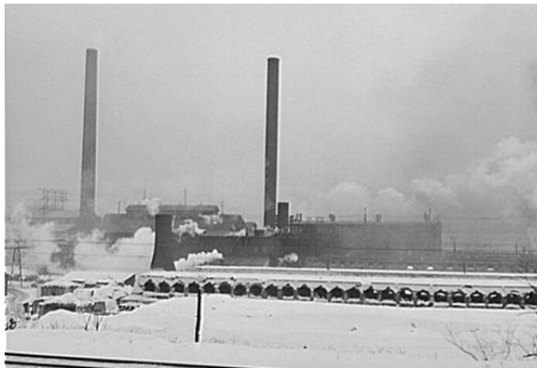
FIGURE 7: Beehive coke ovens in front of steel mill, Aliquippa, Pa., 1941. The roasting of bituminous coal in Pennsylvania's beehive coke ovens, more than 46,000 of which were operation in the 1910s, poured huge clouds of toxic smoke into the air twenty-four hours a day, 365 days a year. The chemical cocktail of tar, benzene, lead, sulfur dioxide, and more than a thousand chemical compounds poisoned the surrounding landscape and caused untold illnesses among coke workers and residents of Pennsylvania coal country. Courtesy of the Library of Congress.
