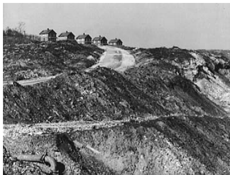
FIGURE 15: Slag piles beneath company town near Montour No. 4 mine of the Pittsburgh Coal Company, Washington County, Pa., 1942. Pennsylvania's iron furnaces produced a huge volume of molten slag—impurities that separated from iron during the smelting process—which was drained out of the furnace, cooled into solid pieces, and then dumped, sometimes piling into huge mounds. Courtesy of the Library of Congress.
