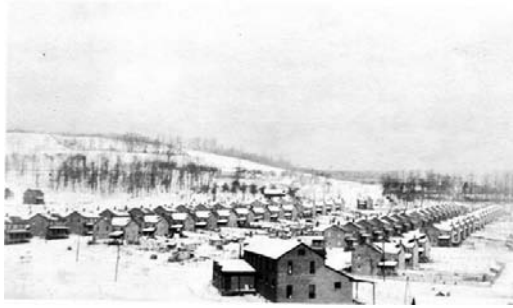
FIGURE 11: Company-owned housing near Eureka Mine 37, Windber, Pa., circa 1920. This winter photograph of housing owned by the Berwind-White Coal Company captures the isolation of the coal-patch towns erected by mine companies during the coal boom of the nineteenth and early twentieth centuries. Courtesy of the Special Collections and University Archives at Indiana University of Pennsylvania.
