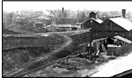
Figure 16. Looking southwest from the corner of Biddle and Adams Streets. The connecting track disappears to the right behind part of the Sharples Separator Works, while a siding curves up and over Chestnut Street into the Hemphill lumber yard. The HBD smokestack is visible beyond the siding. Photo by Albert Biles, ca. 1899, courtesy of the Chester County Historical Society, West Chester, PA.
