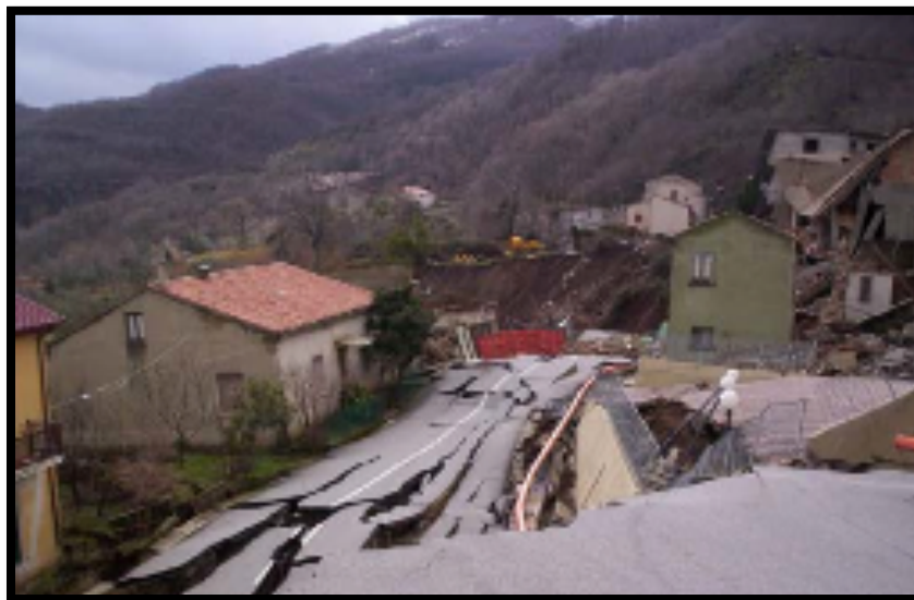
Photo 2: The Emigrants’ Road after the landslide
