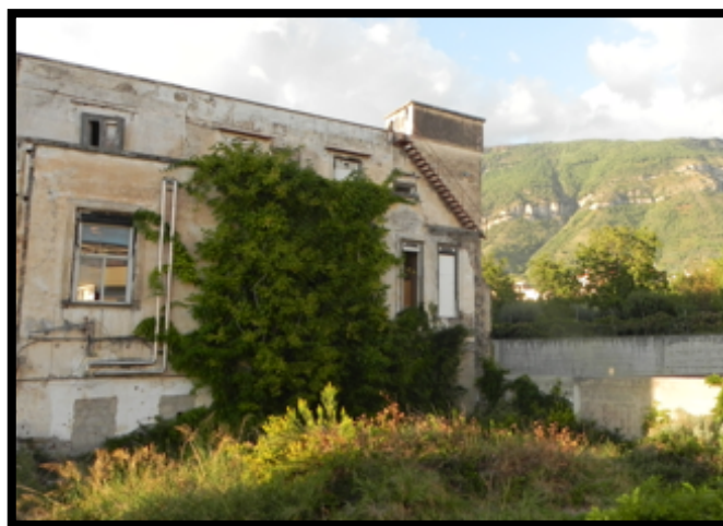
Photo 9: The Villa Malta hospital in 2012
