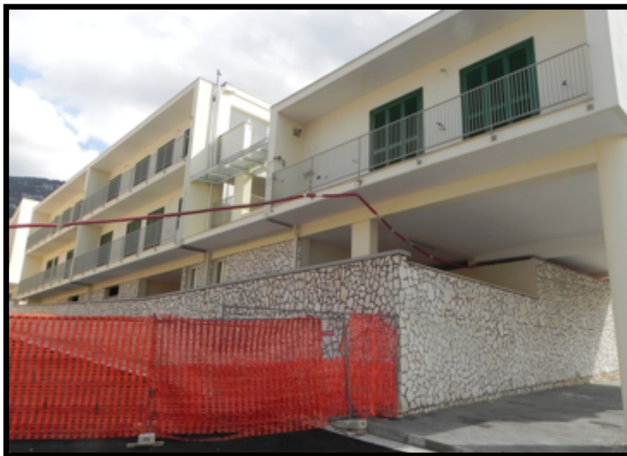
Photo 18: Housing projects in Via Episcopio, under construction
