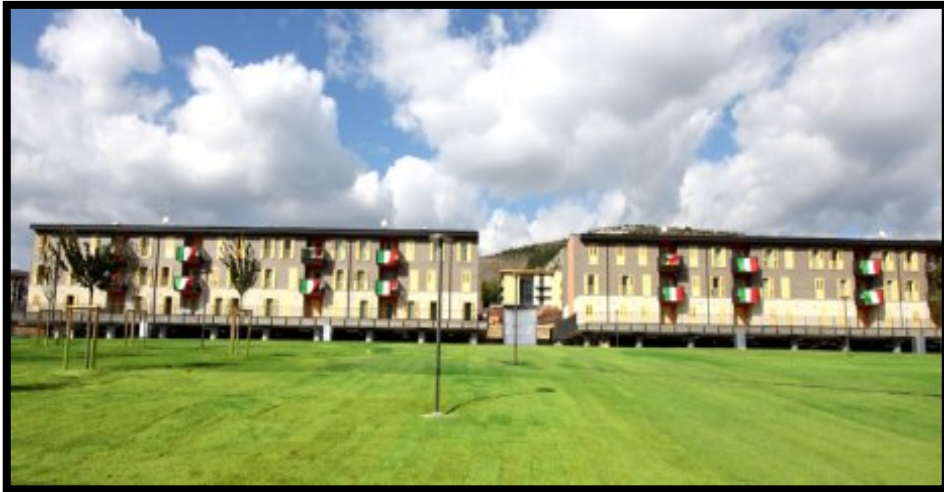
Photo 23: The new buildings in the “new” Aquila
