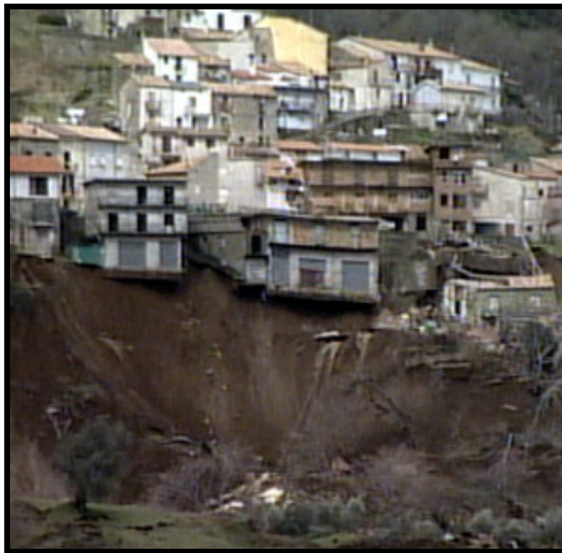
Photo 5: The Cerzeto landslide in the Cavallerizzo district
