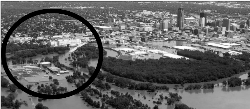
Figure 5: Water Works and the 1993 Flood 56
