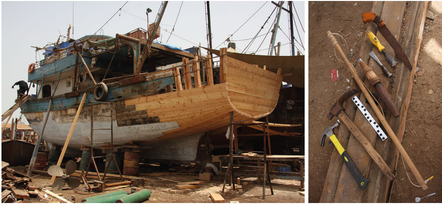
Fig. 5 Left An ‘Egyptian’-style fishing sanbūk under repair at the yard of Ibrahim Bilghaith. Right The tool kit of the wooden-boat builder (Images: J. P. Cooper)
