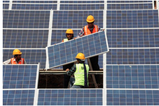
Installation of Rooftop DG Facility
