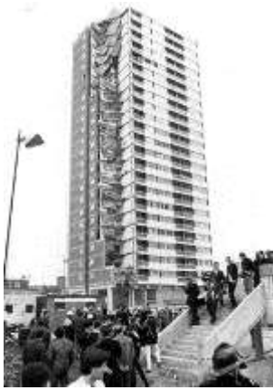
Figure 2 Ronan Point partial collapse, Source: Wikipedia, Image rights "London Over the Border" [1], a historical website produced by the London Borough of Newham. Image is credited to The Daily Telegraph, 1968
