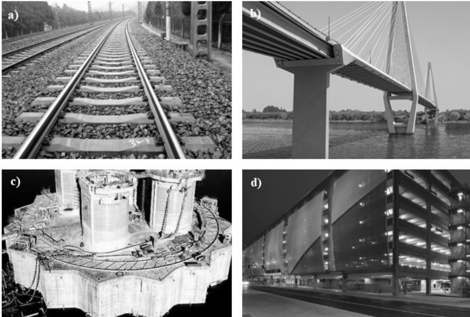
Fig. 1.1. Prestressed concrete structures undergoing fatigue effect: a) concrete sleepers (You et al. 2017); b) bridges; c) offshore oil platforms; d) parking garages (Cleland et al. 2015)
