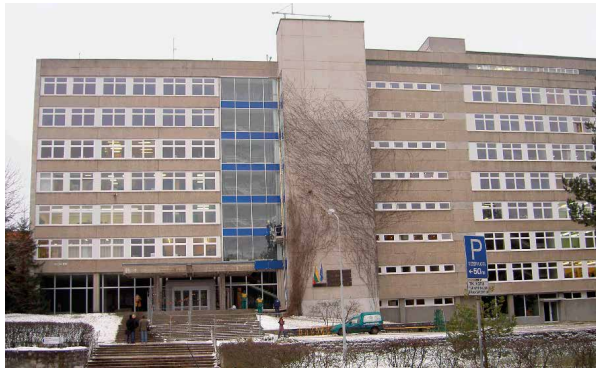
Figure 3.13. A view of the main building of VGTU with replaced windows
