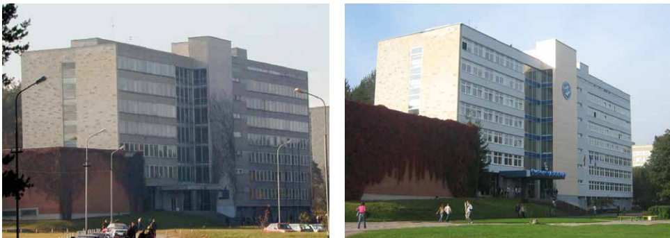
Figure 3.10. The main building of Vilnius Gediminas Technical University before and after retrofitting
