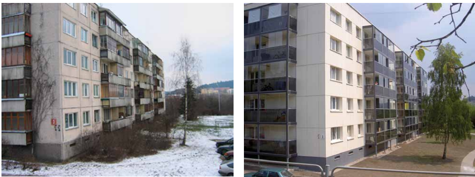
Figure 3.9. A panel house in Vilnius, Zirmunai St. 3, before and after retrofitting based on a package of basic investments
