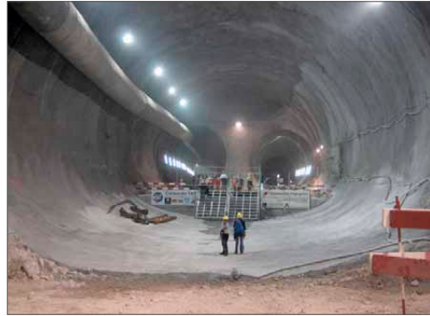
Figure 20.12. The Gotthard Base Tunnel in Switzerland: a – the tunnel boring machine breaking through rocks; b – tunnel junction at a multifunction station
