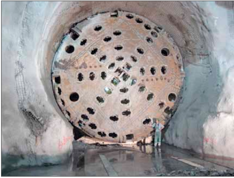
Figure 20.12. The Gotthard Base Tunnel in Switzerland: a – the tunnel boring machine breaking through rocks; b – tunnel junction at a multifunction station
