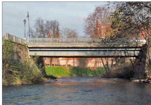
Figure 19.1. A beam bridge
