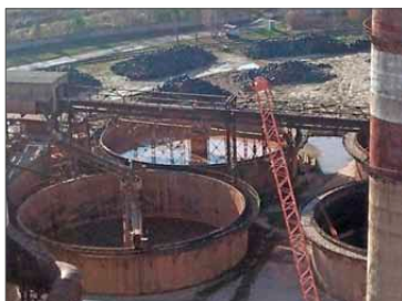
Figure 24.3. The cement manufacturer in Naujoji Akmenė: a – circular slurry mixer basins of plants using the wet process, b – general layout of a rotary kiln
